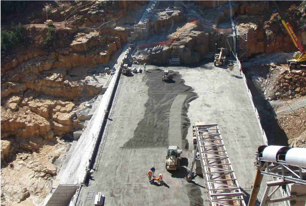
Figure 2-4 Typical RCC dam construction with concrete conveyor
