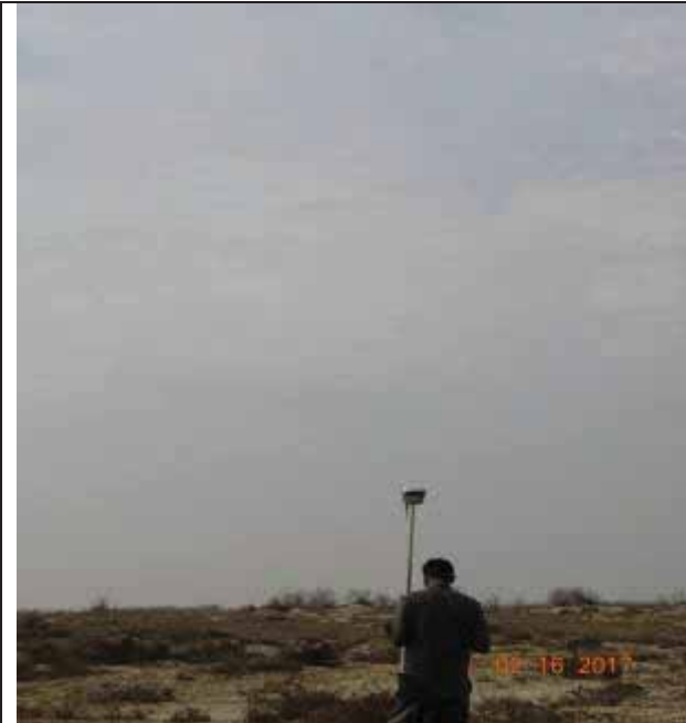
Site survey for Geotechnical Investigation
