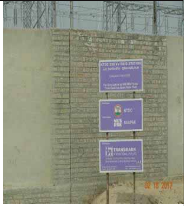
220kv NTDC Grid in QASP
