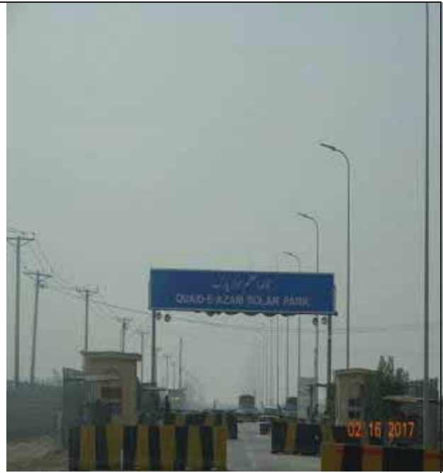
QASP Entry Point
