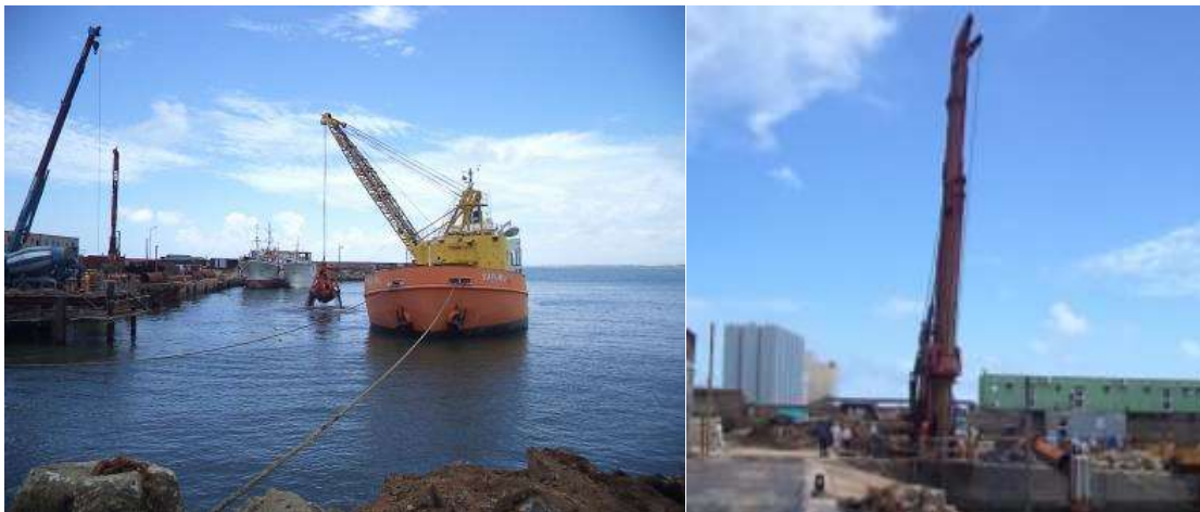
Photo 1: View of Dredger and Piling Equipment
