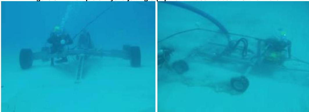
54. The hydro-jetting technique is anticipated to have the least environmental impact in the nearshore marine environment (J. Hibbard, 2015 Pers. communication). Hydro-jetting is useful in applications where seabed materials are consolidated. Hydro-jetting is proposed to be undertaken in submarine areas up to 200m depth (in some cases involving remotely controlled plows). Beyond this depth, the cable will be laid on the sea floor without the need for trenching.
