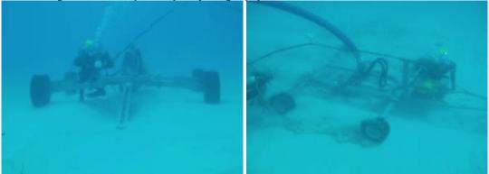
54. The hydro-jetting technique is anticipated to have the least environmental impact in the nearshore marine environment (J. Hibbard, 2015 Pers. communication). Hydro-jetting is useful in applications where seabed materials are consolidated. Hydro-jetting is proposed to be undertaken in submarine areas up to 200m depth (in some cases involving remotely controlled plows). Beyond this depth, the cable will be laid on the sea floor without the need for trenching.
