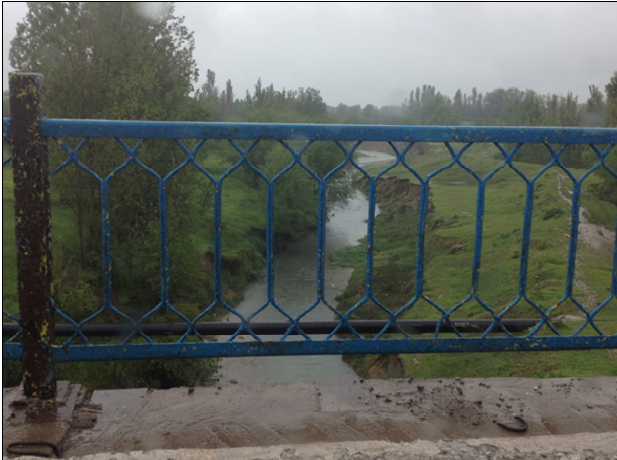
Figure D.5: Aksudarya river (Km 106)
