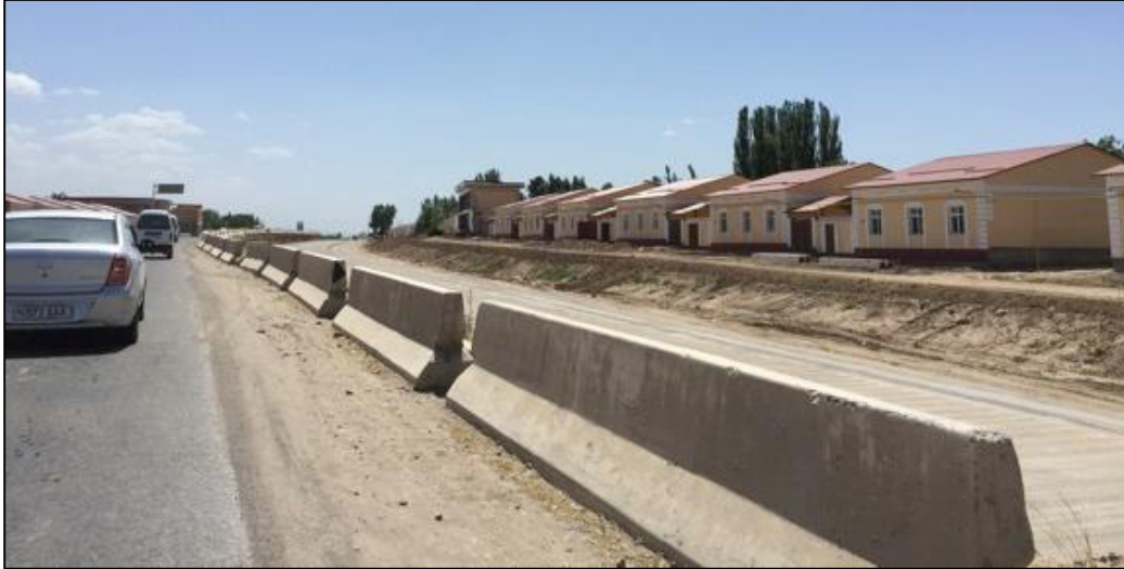
Figure E.2: Construction works have limited access to the opposite side of the road.
