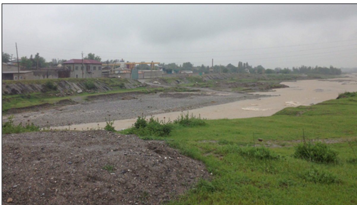
Figure D.4: Kashkadarya River (km 113)
