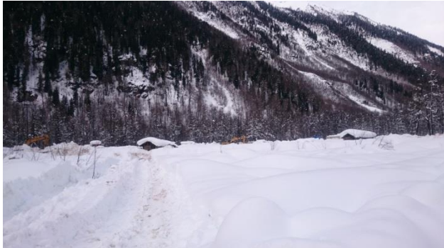
Figure A.23: Dam site area from the distance with the two wooden sheds
