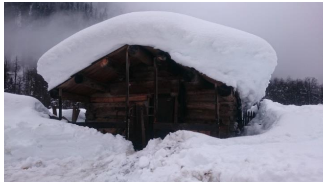
Figure A.22: Wooden shed on dam site area
