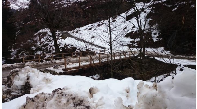
Figure A.2: Bridge N2
