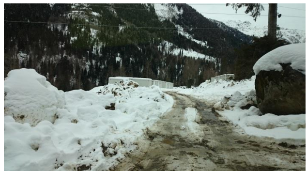
Figure A.4: EPC Contractor Temporary Construction Offices – not in use at time of site visit
