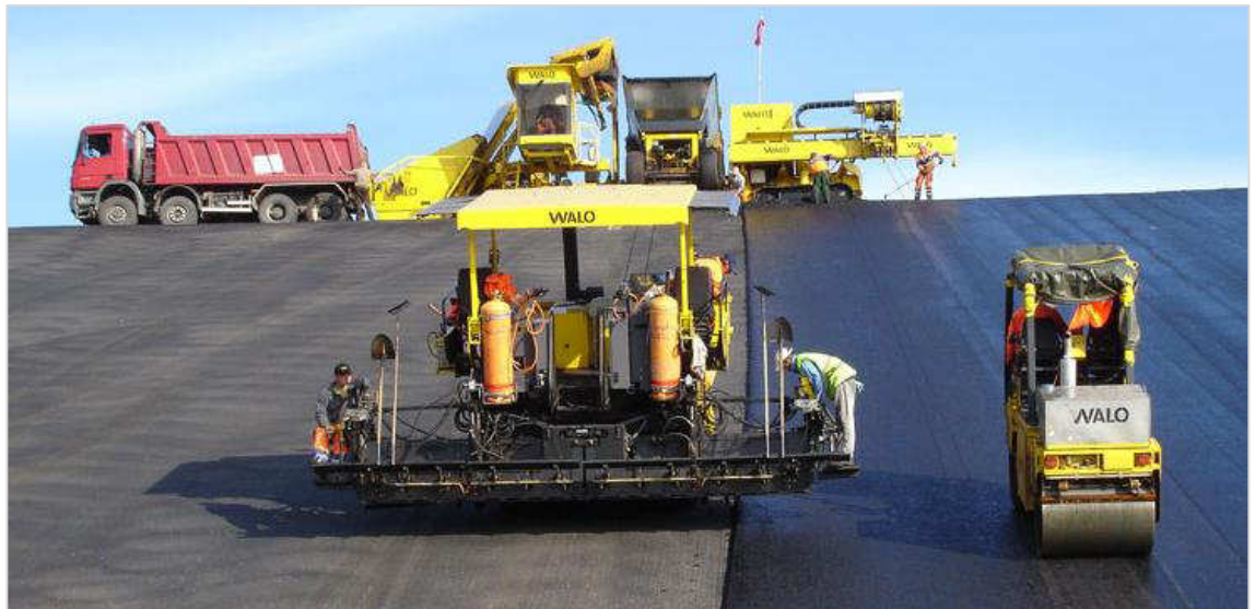
Figure 45 - Illustration of asphalt paver on dam face
