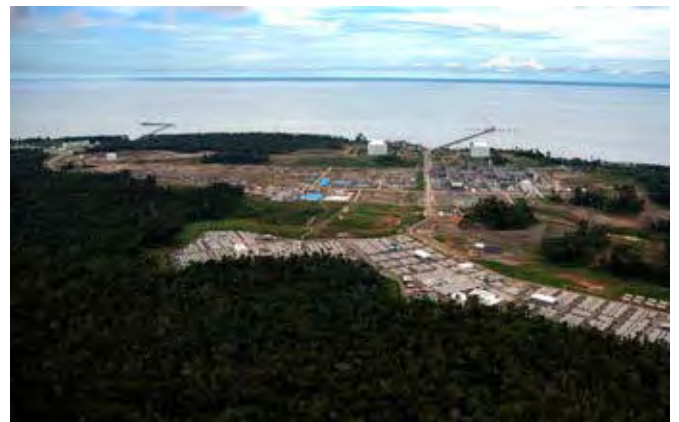
Figure 6 Facilities within Tangguh LNG site
