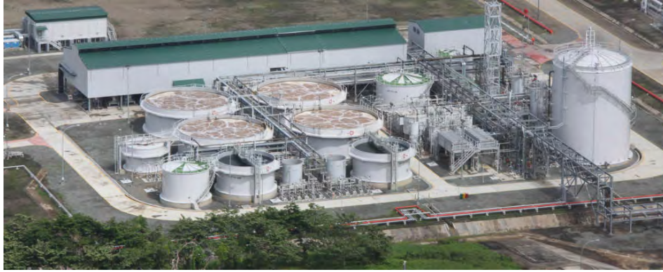
Figure 23 Produced Water Treatment Plant
