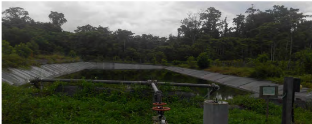
Figure 20 High water level in new landfill leachate pond
