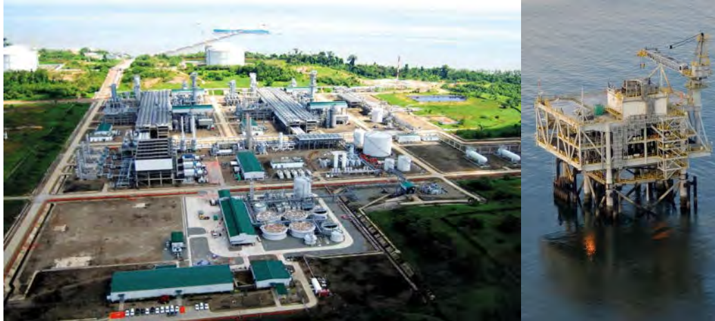
Figure 11 Aerial View of Tangguh T1/2 onshore facilities and VRA Platform
