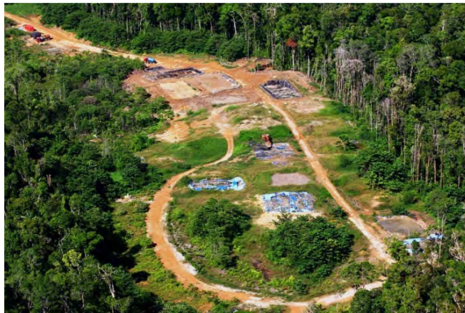
Figure 3 Organic Waste Pits during T1/2 Construction Phase (2009)
