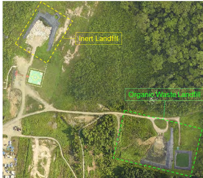
Figure 4 Aerial View of Inert and Organic Waste Landfills
