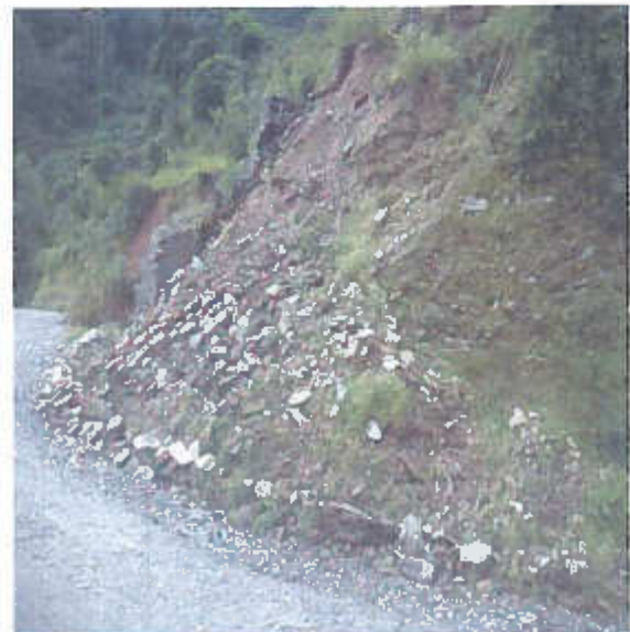
Plate 10: Minor Slide at Ch. 6+350
