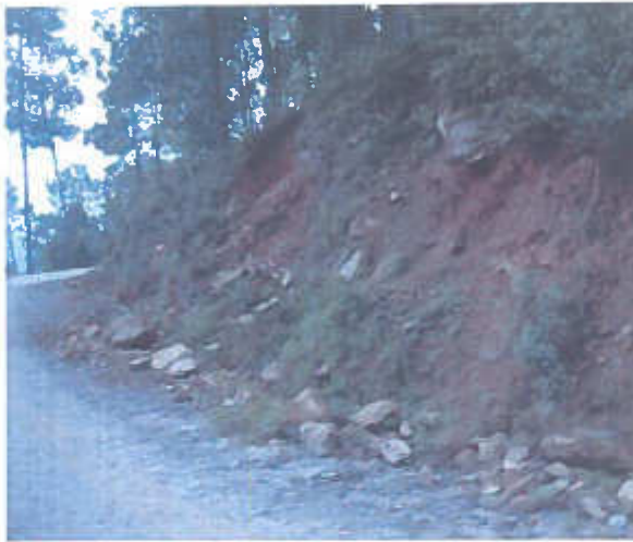
Plate 18: Minor Slide at Ch. 24+280
