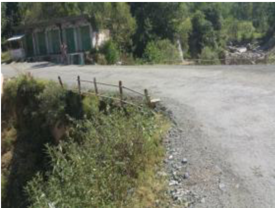
Bridge Near village Piya on Kalam Road Madyan to be reconstructed
