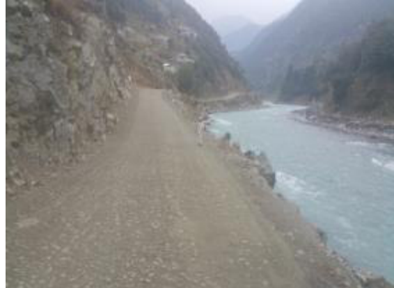
Behram-Kedam Road section to be reconstructed
