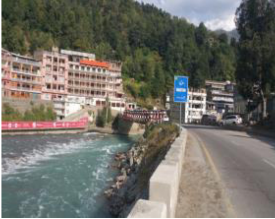
Satal Village and River Swat adjacent to Madyan Bridge to be reconstructed
