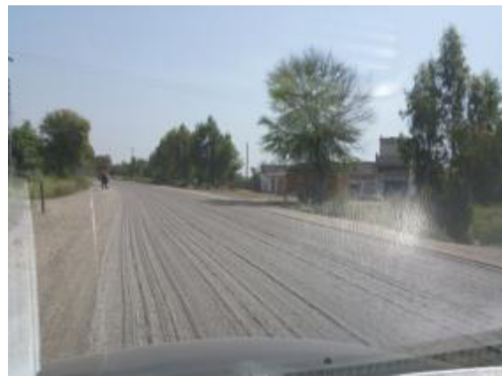
Kohat-Karak Road section to be rehabilitated
