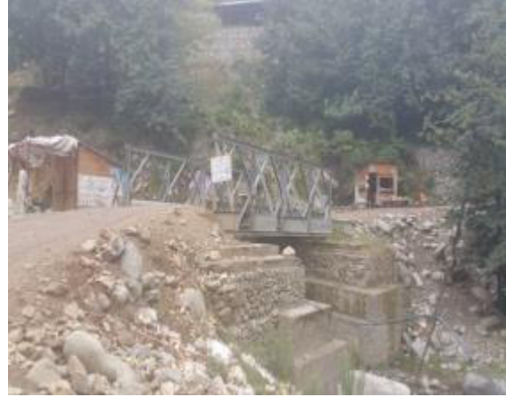
Cham Garhi Bridge Kalam Swat and road section to be reconstructed
