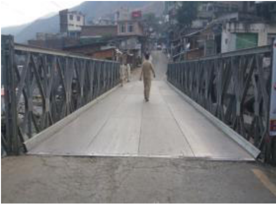
View of Existing Bahrain Bridge in Swat to be reconstructed
