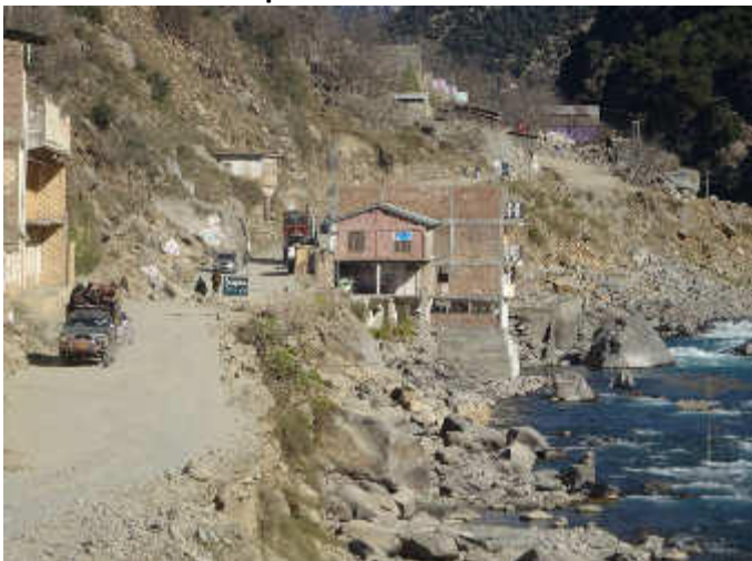
Pkg 1, Lot 1, RD 99+100 to 99+300: commercial structures located on left side of existing carriageway but have no LAR impacts.
