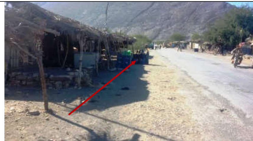
Pic. 2 (1) Lot-1 N-50: Mughalkot Temporary structures located out of shoulder edge on right side of road. N-50_RD 395+550 to RD 395+600
