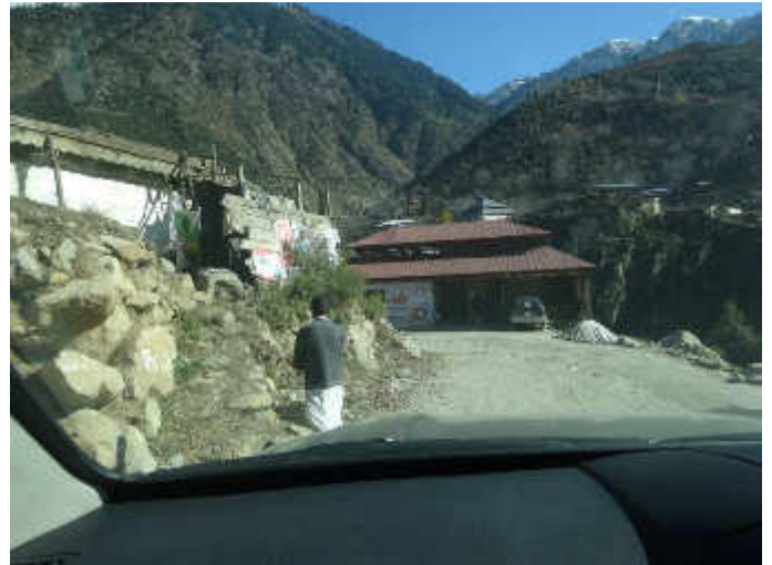
Pkg 1, Lot 2, RD 109+210. Six commercial structures encroaching the existing working space of about 6m.
