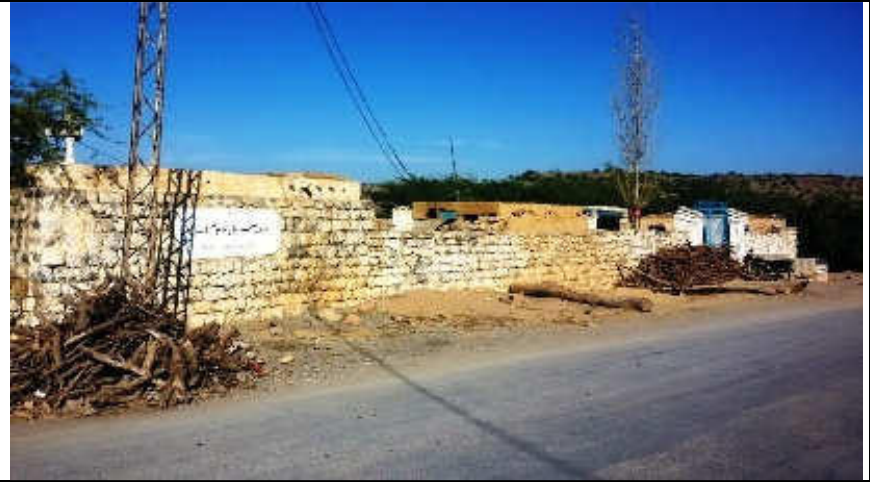
Pic. 7 (2) Lot-1 N-50: Madrsa (traditional institute for religious education) located out of existing carriageway shoulder on right side of road (front view). N-50_RD 425+200
