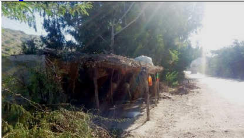
Pic. 5 (1) Lot-1 N-50: Shop with extended shed located out of existing carriageway shoulder on left side of road. N-50 RD 419+000
