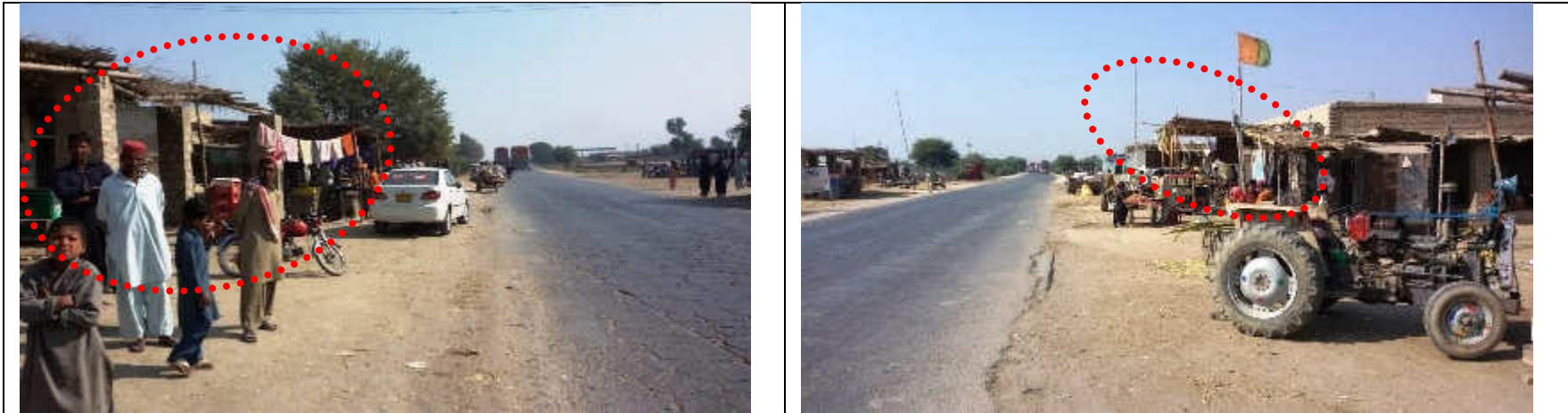
Pic.6 (2) Lot-1 N-55: Encroached temporary structures (sheds and kiosks along both sides of existing carriageway but outside of earthen shoulder (road side view). N-55_RD 477+800 to RD 477+900
