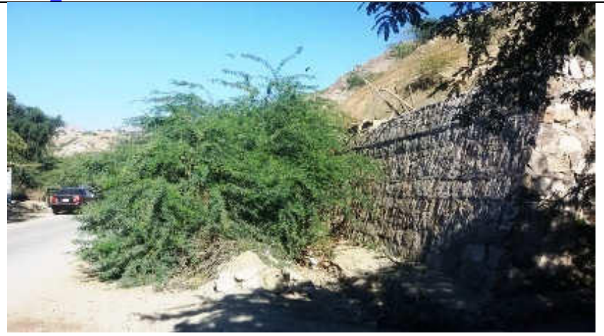
Pic. 5 (2) Lot-1 N-50: Stone masonry wall out of existing carriageway shoulder on right side of road. N-50 RD 419+000 to 419 +100
