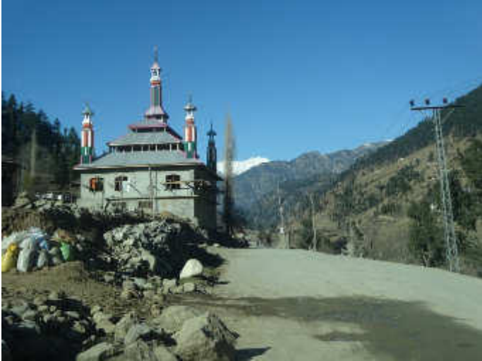
Pkg I, Lot 3 RD 125+610. Mosque clear from existing carriageway. No impacts.
