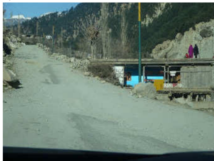
Pkg 1, Lot 3, RD 120+600, Residential/commercial structures encroaching the existing working space of 8-10m
