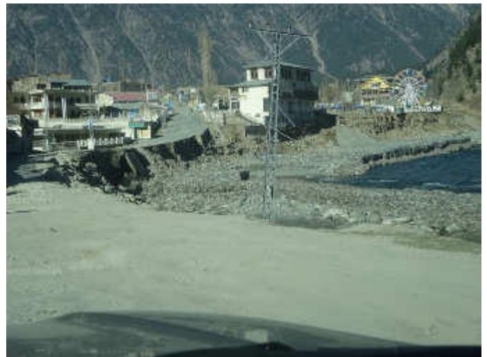
New alignment of 300 m under construction near end point of Kalam but no LAR impacts
