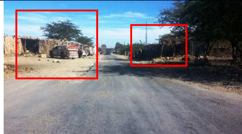
Pic. 1 (2) Lot-1 N-50: Mughal kot encroached road section (Zhob Side view) showing that only carriageway is clear in this section and structure on left are within shoulder limit. N-55_RD RD 395+500 to 395+550
