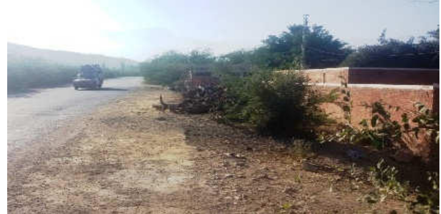
Pic. 1 (2) Lot-2 N-50: Residential Structures located out of existing carriageway shoulder on right side of road. N-50_RD 449+000
