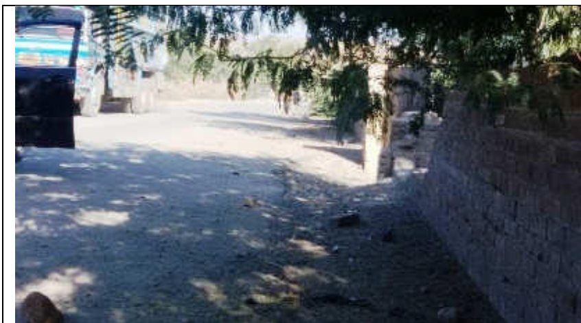
Pic. 8 (1) Lot-1 N-50: Boundary wall of NHA owned structure (abandoned lab) located out of existing carriageway shoulder on left side of road (side view). N-50_RD 425+900
