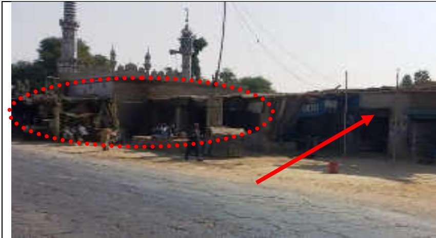
Pic.5(3) Lot-1 N-55: Shops at edge of ROW showing encroachments like mosque with temporary sheds along right side of existing carriageway. N-55 RD 477+800 to RD 477+900
