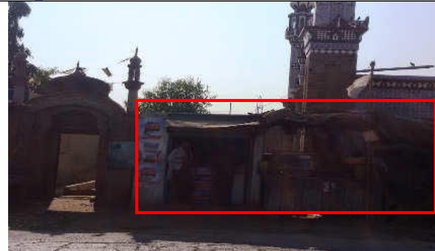
Pic.5(2) Lot-1 N-55: Mosque wall with brick masonry shop and thatched sheds located on earthen shoulder along right side of existing carriageway (front view). N-55_RD 477+800 to RD 477+900
