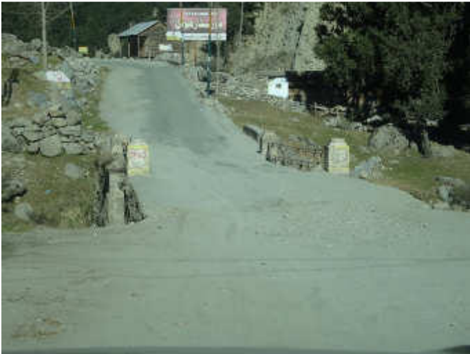
Pkg 1, Lot 3, RD 121+510, One residential structure touching the carriageway from left side. Keep construction within 10m to avoid impacts.
