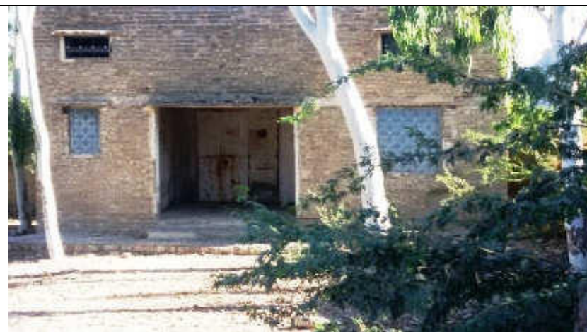
Pic. 8 (2) Lot-1 N-50: Front view of NHA owned structure (abandoned lab) located out of existing carriageway limits but boundary wall is adjacent to shoulder. N-50_RD 425+900
