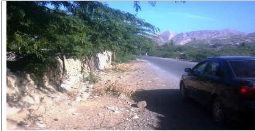
Pic. 3 (1) Lot-2 N-50: Residential Structures located out of existing carriageway shoulder on left side of road (Aman Kaley village). N-50_RD 449+300 to 449+500
