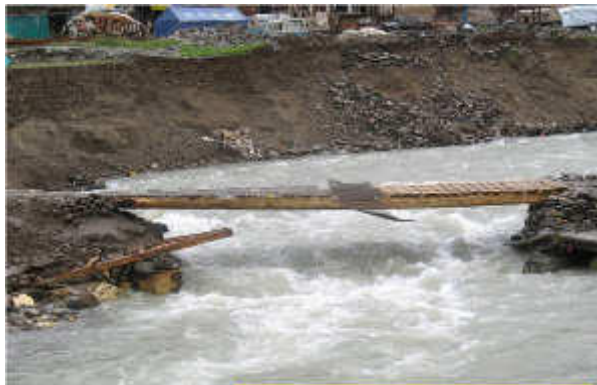
Wooden bridge spanned at Batakundi Km 151, N-15
