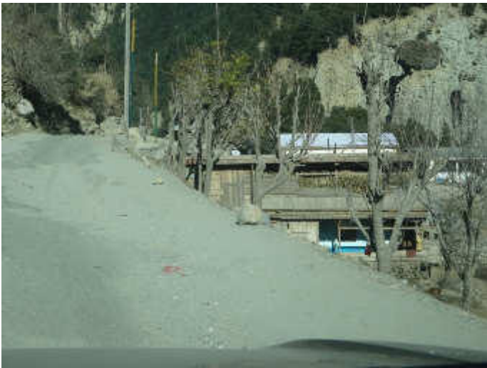
Pkg 1, Lot 3, RD 121+510, One residential structure touching the carriageway from left side. Keep construction within 10m to avoid impacts.
