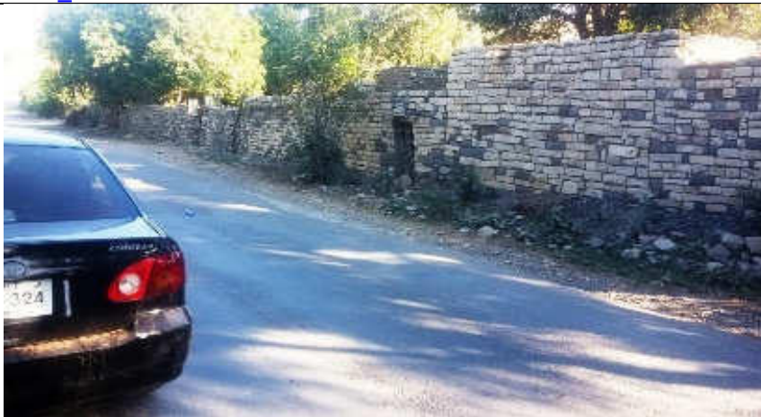
Pic. 2 (1) Lot-2 N-50: Residential Structures located at edge of existing carriageway shoulder on right side of road (Aman Kaley village). N-50_RD 449+300 to 449+500
