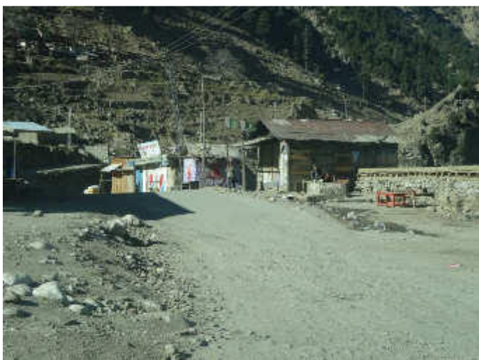
Pkg 1, Lot 2, RD 116+900, About 20 commercial structures encroaching upon the existing working space of about 8-10m.
