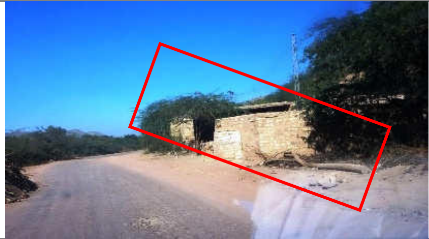
Pic. 4 (2) Lot-1 N-50: Residential Structures located out of existing carriageway shoulder on right side of road (road side view) Village Ghal Kaley. N-50 RD 415+000 to 415 +100
