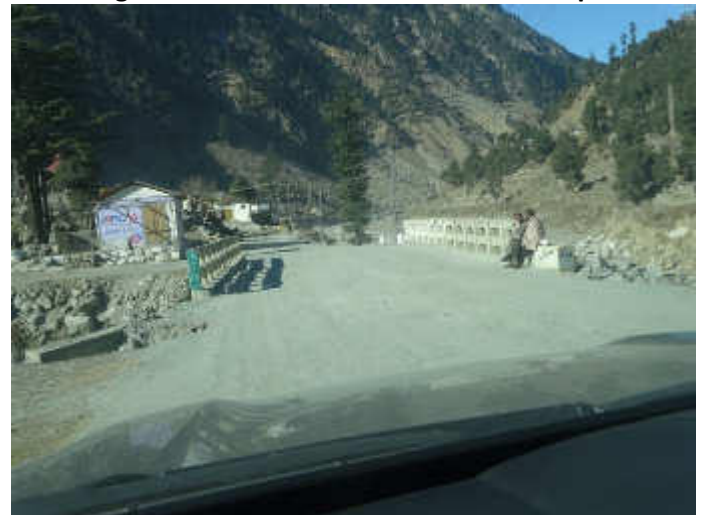
Pkg 1, Lot 3, RD 121+110: Six residential structures
