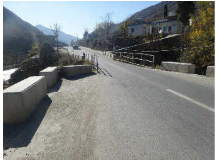
Pkg-I, Lot 1, Bridge at RD: 91+520
