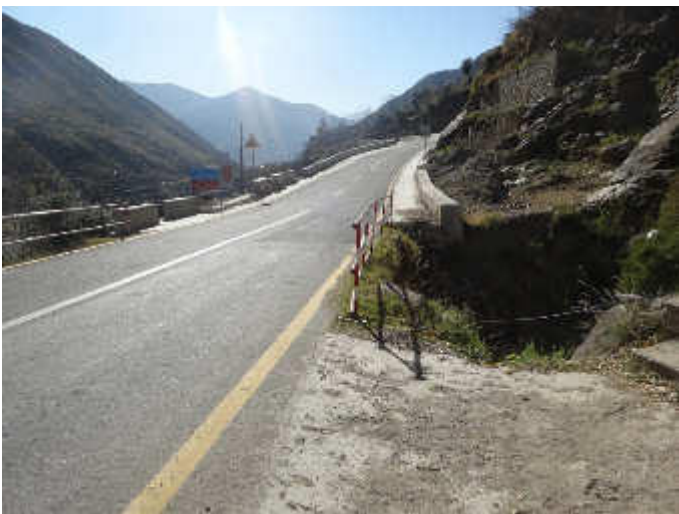
Pkg-I, Lot 1 Satal Bridge at RD: 92+190
