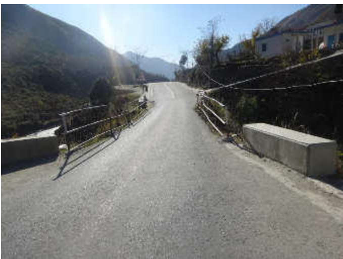
Pkg-I, Lot 1, Bridge at RD: 91+520
