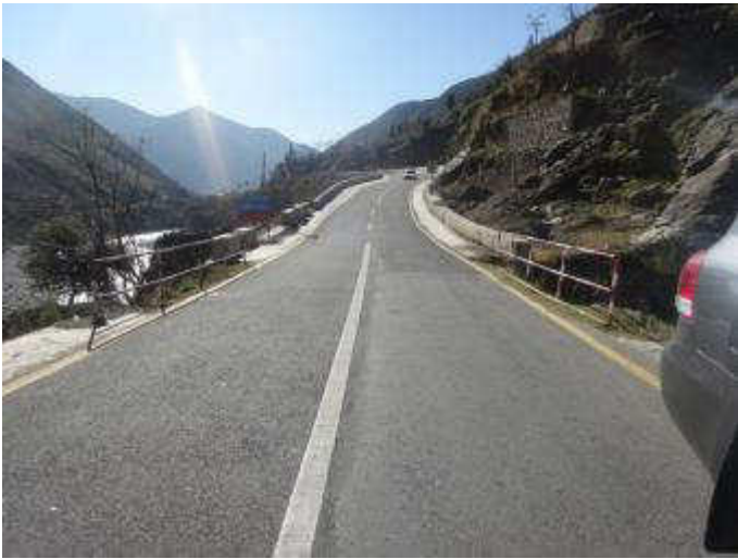
Pkg-I, Lot 1 Satal Bridge at RD: 92+190
