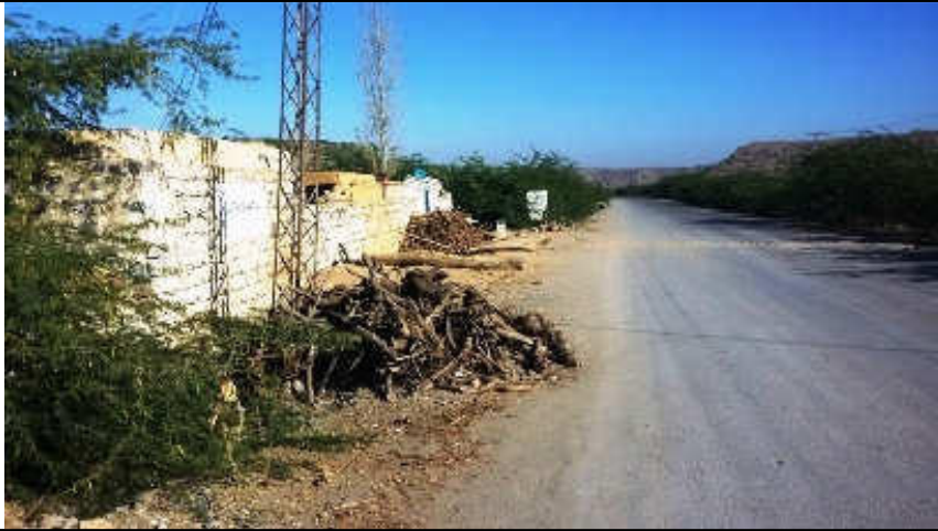
Pic. 7 (1) Lot-1 N-50: Madrsa (traditional institute for religious education) located out of existing carriageway shoulder on right side of road (side view). N-50_RD 425+200
