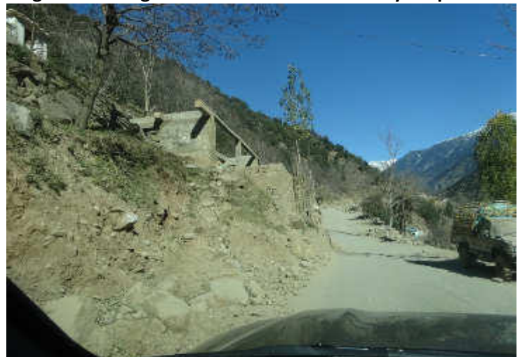
Pkg-I, Lot 1, Structures near bridge at RD: 101+095. Restrict construction within 10m to avoid impacts
