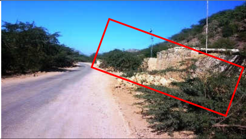
Pic. 4 (2) Lot-1 N-50: Residential Structures located out of existing carriageway shoulder on right side of road (road side view) Village Ghal Kaley. N-50 RD 415+000 to 415 +100
