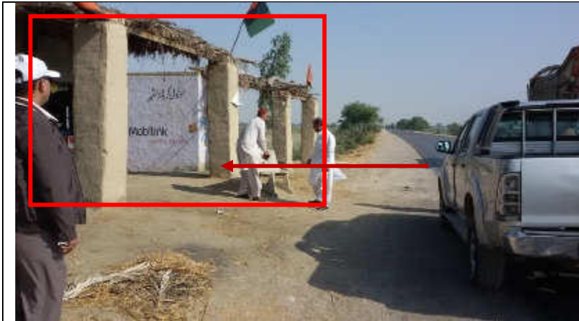
Pic. 3 Lot-1 N-55: Brick masonry Structure (shops) with shed (left side) located out of existing carriageway shoulder. N-55_RD 473+700
