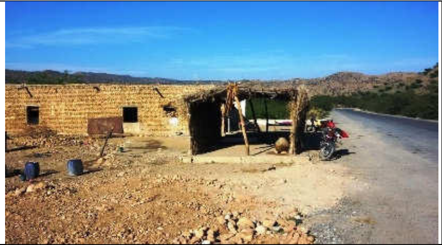
Pic. 6 (2) Lot-1 N-50: Shop with extended shed located at outer edge of existing carriageway shoulder on right side of road. N-50_RD 425+200
