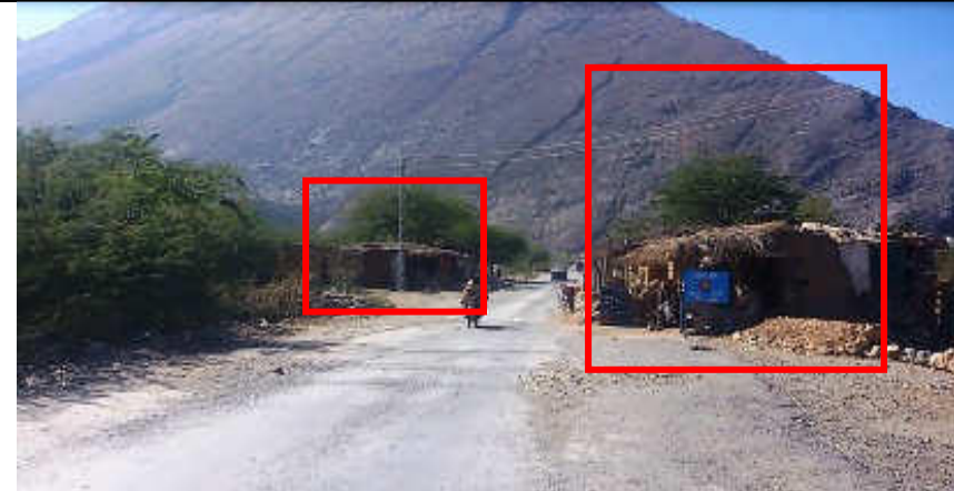
Pic. 1 (1) Lot-1 N-50: Mughal kot encroached road section (DI Khan side view), structure on right side are shown on shoulder limits. N-50_RD 395+500 to 395+550
