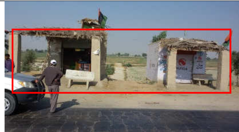
Pic. 4 Lot-1 N-55: Front view of brick Masonry Structure (shops) with shed (leftt side) N-55_RD 473+700
