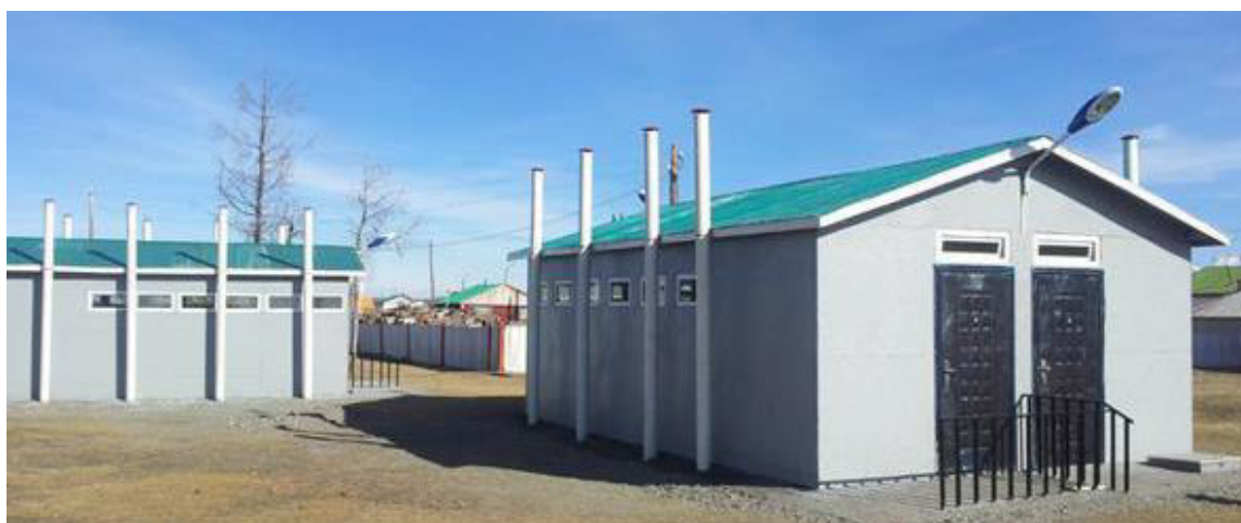
Figure 2: Example of Ventilated Improved Pit Latrines applied for schools in unsewered areas of Mongolia, supported by UNICEF, Mongolia (2014).
