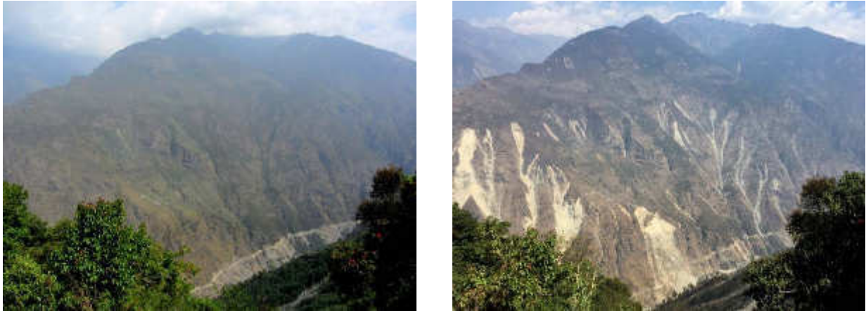
Figure 1-3: Trishuli Canyon and Access Road Before and After the April 2015 Earthquake
