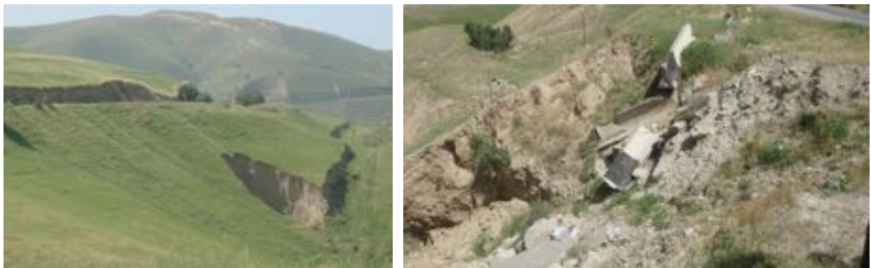
Fig. 12: Challenging soil characteristics aggravated with improper drainage give rise to rapid damage to road structures at several locations
