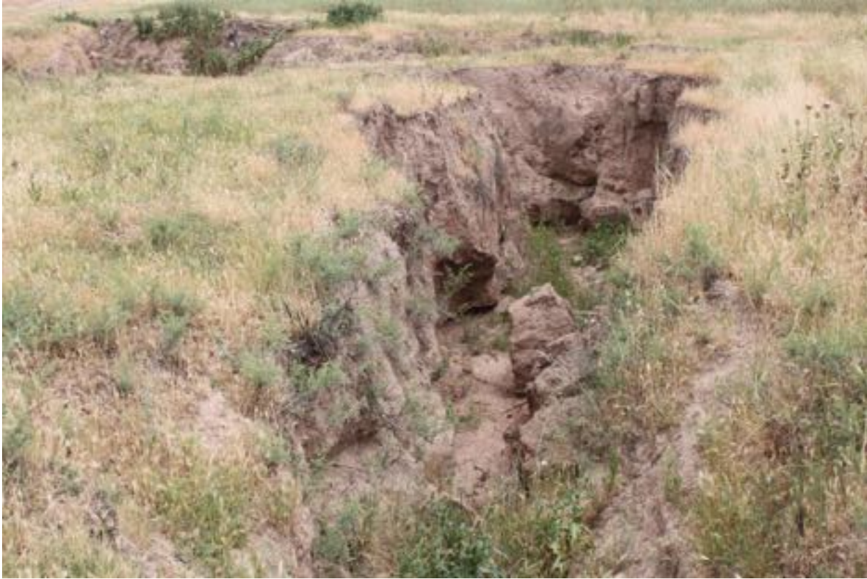
Fig. 22: Gully erosion alongside the Project Road
