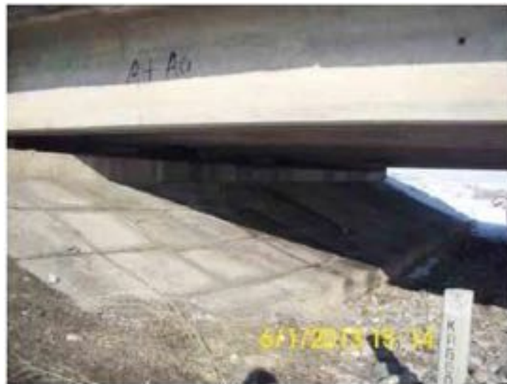
Fig. 25: An example of bridge slope protection
