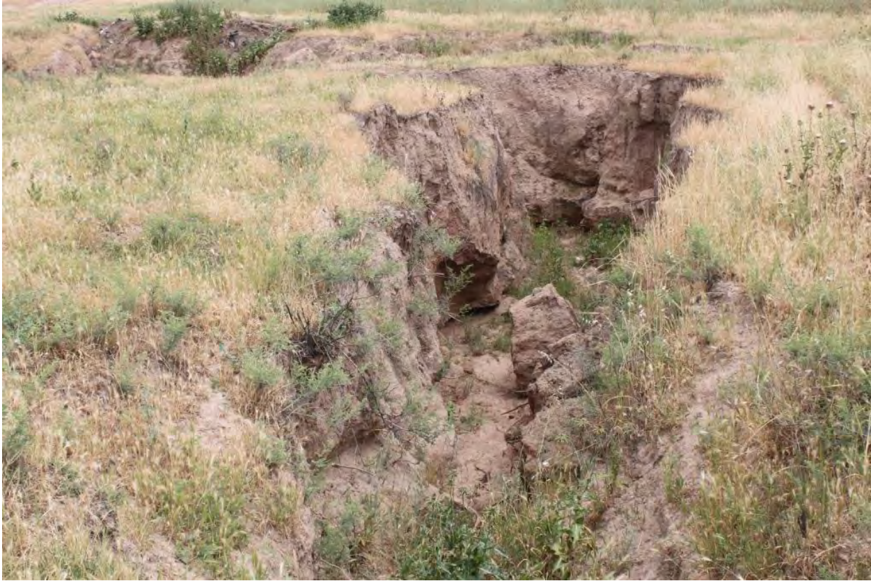
Fig. 17: Gully erosion alongside the Project Road
