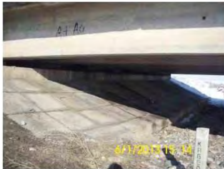
Fig. 20: An example of bridge slope protection
