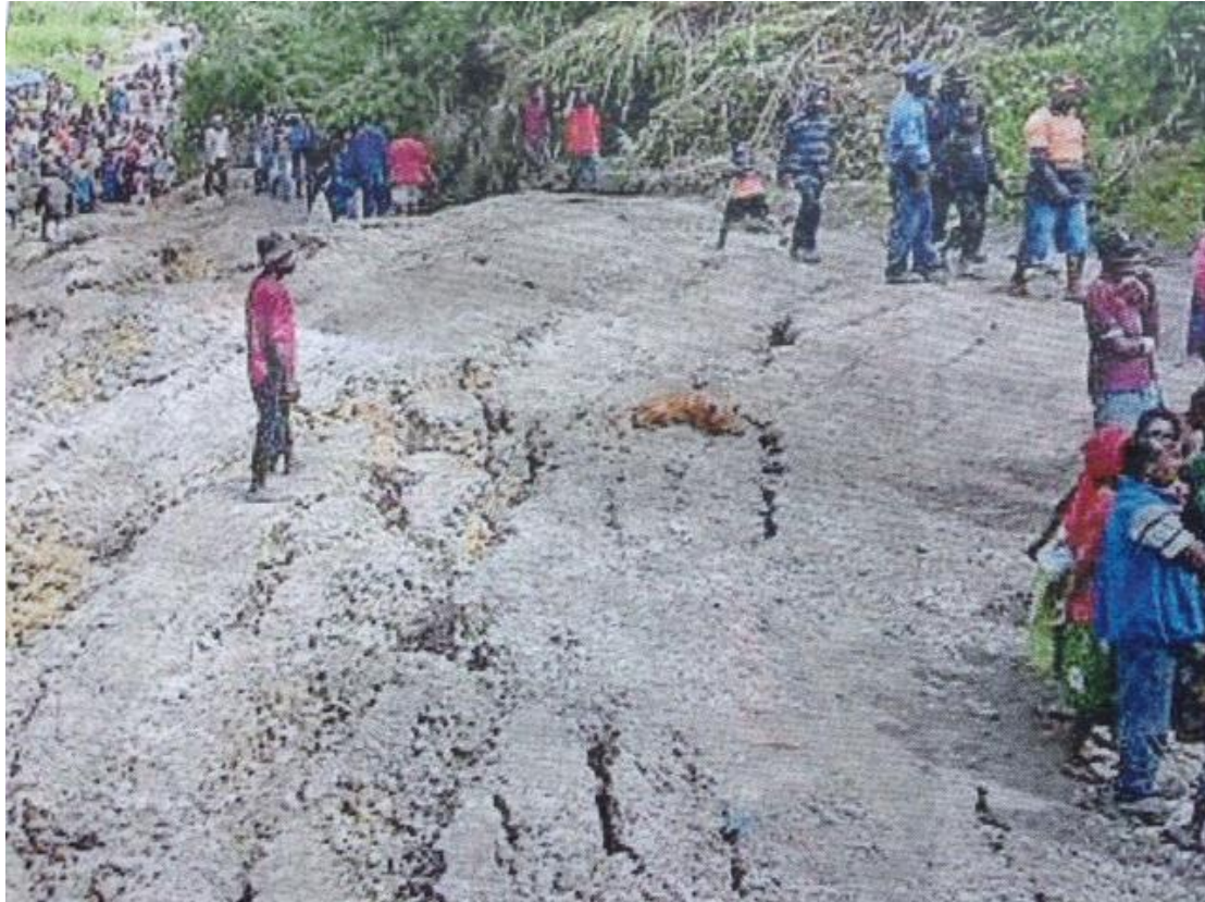
Newspaper photograph of the damaged road, before the landslide in January 2017
