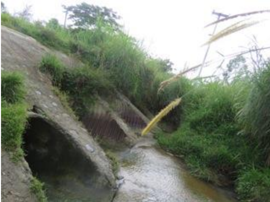
One of the large five-channel culverts at each end of the damaged road section
