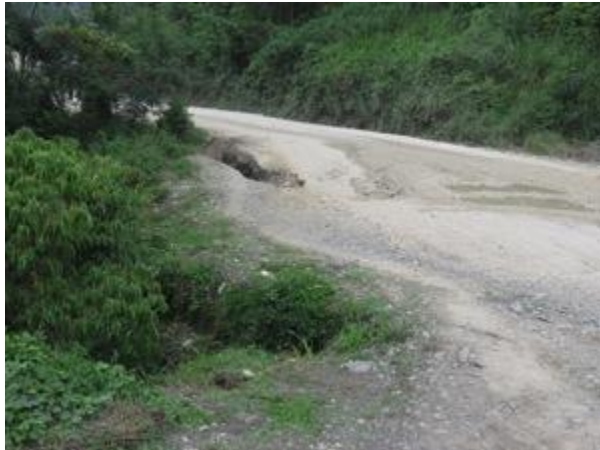
Guo: Severe regressive erosion, surface water, deep holes and drainage problems on slopes
