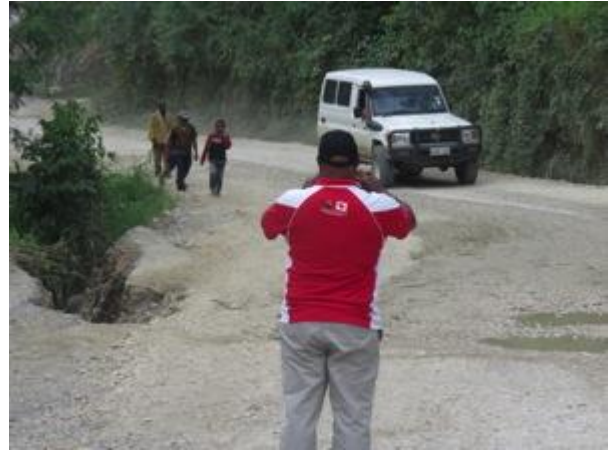
Guo: Severe regressive erosion, surface water, deep holes and drainage problems on slopes
