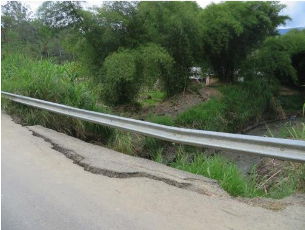
Ba Creek, showing collapsed road edge and blocked culvert
