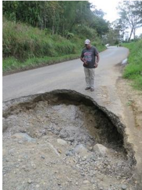
An unreported collapse of the road near Yonki
