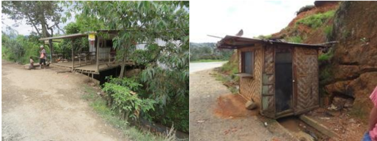
Structures built on top of road drainage channels, which can cause blockages
