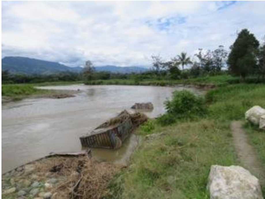
Remaining stone-filled containers put in to protect river bank
