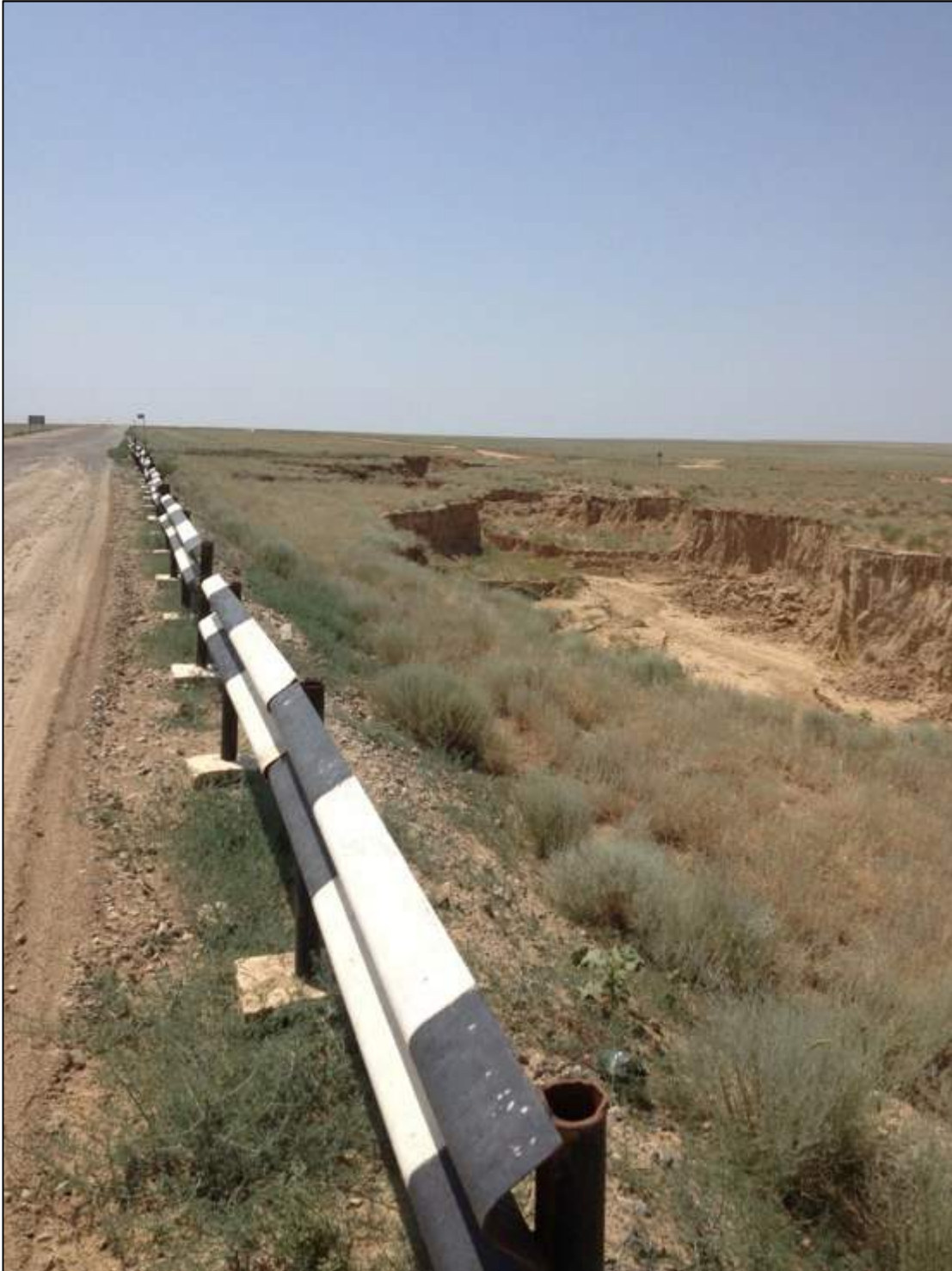
KM+347: Safety barriers have been placed adjacent to this gully to prevent drivers crashing into the gully if they fall asleep at the wheel.
