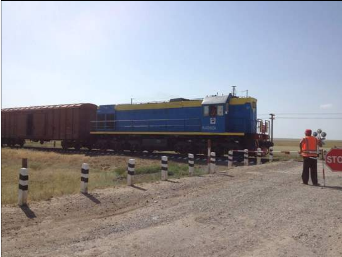
KM+242: Rail crossing at Bayganin. The road will be re-aligned here to accommodate an overpass.
