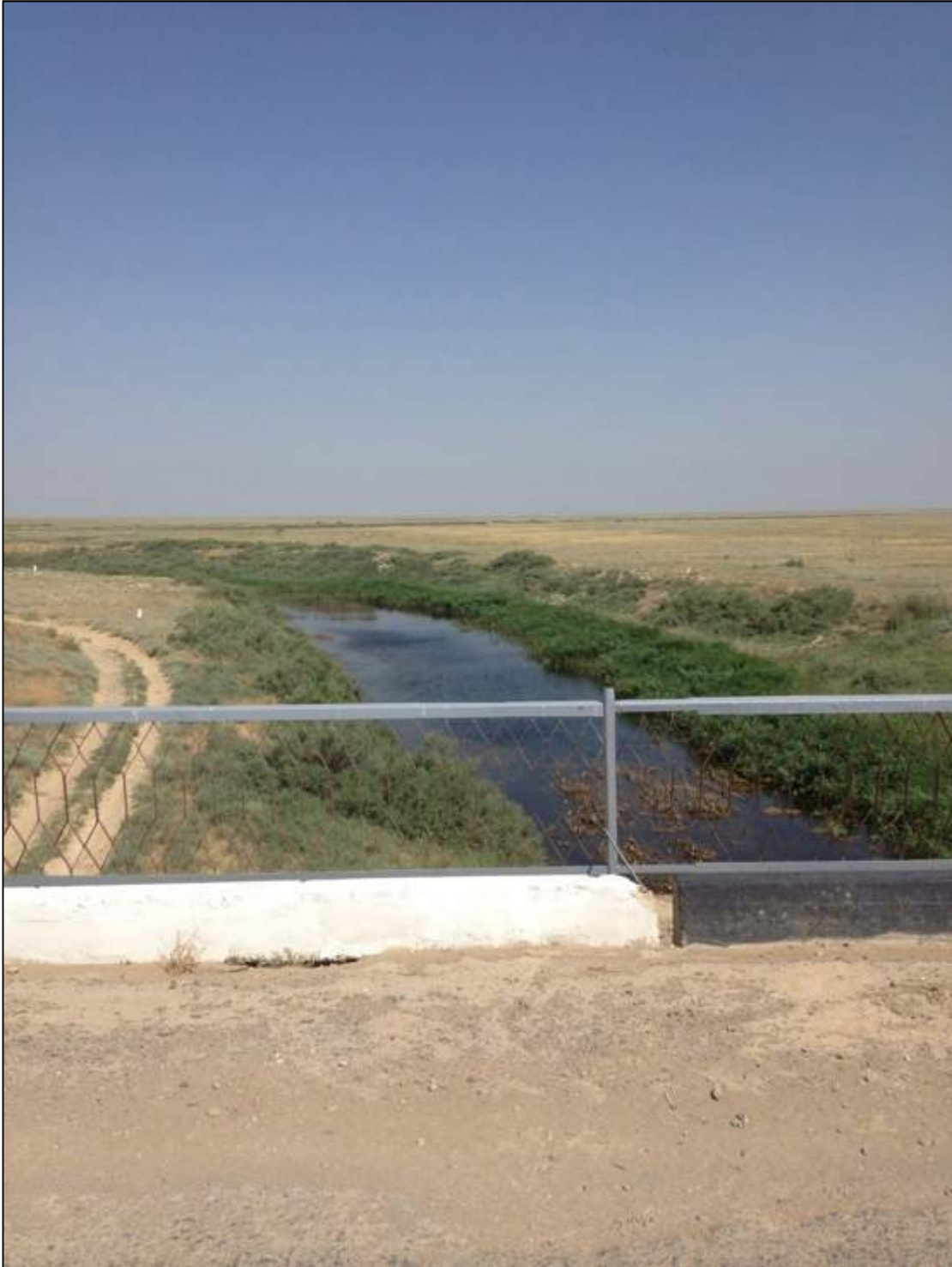
KM+430: This bridge crosses the Sagiz River. The bridge showed signs of aging and the pedestrian pathway appeared to be breaking up. However, due to the remote location of the bridge this pathway would almost certainly never be used.
