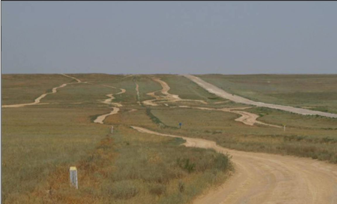
KM+360: The road is the portion furthest to the right of the photo, but due to the poor condition of the road other tracks have been made to bypass these poor sections of road. Accordingly, in this section the road corridor is more than 50 meters wide.
