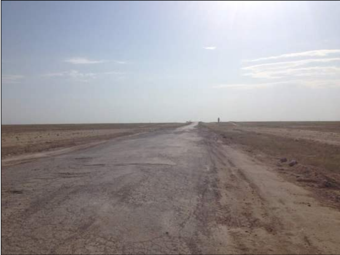
KM+458: Road condition in this area is poor, although portions are asphalted. The road is almost pan flat and traverses desert with little sign of vegetation apart from light grasses. Traffic volume in this section was extremely low, with fewer than two vehicles seen in 30 minutes of driving.
