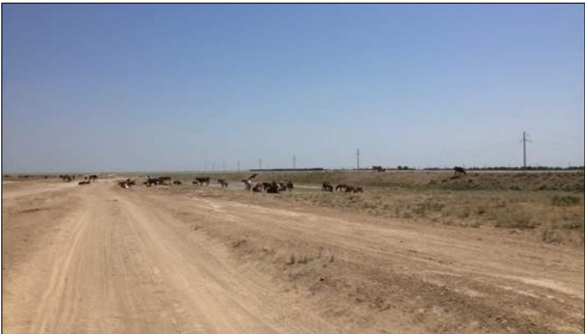
KM+372: Horses and cattle were observed at this section of the road. Animal underpasses will be constructed at locations agreed with by local villagers.
