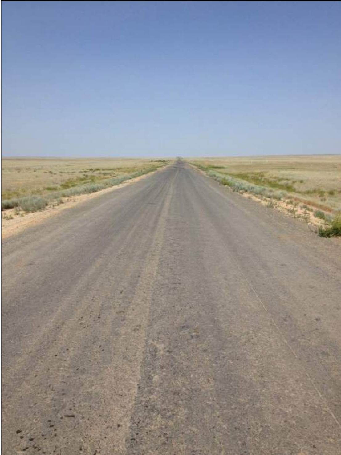
KM+260: A typical road section, straight and flat.
