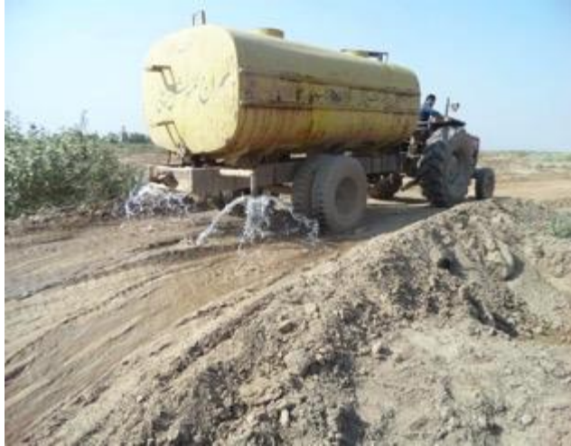
Water is being sprinkled on the service Road to suppress dust
