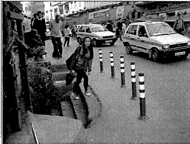
2. Plastic bollards at entrance to public stairs (near City Hospital)
