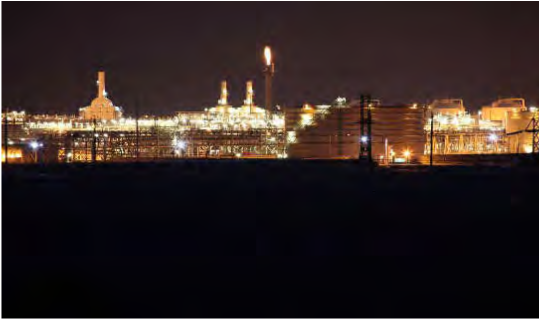
Figure 2.2 Photo from Sangachal Showing Boundary and Plant Lighting of the Terminal
