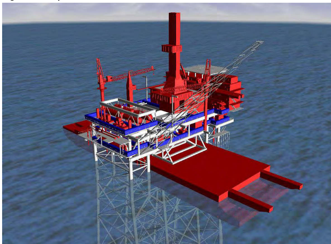
Figure 5.15 Topsides “Float-Over” Installation Method
