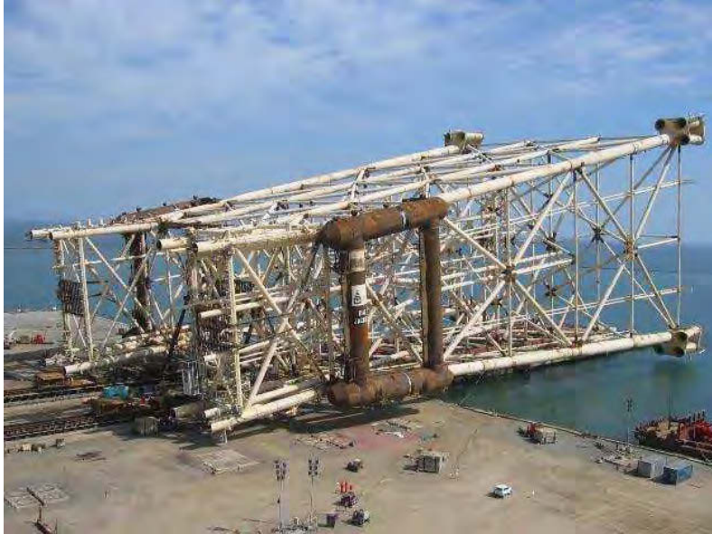
Figure 5.12 DWG-DUQ Jacket During Loadout
