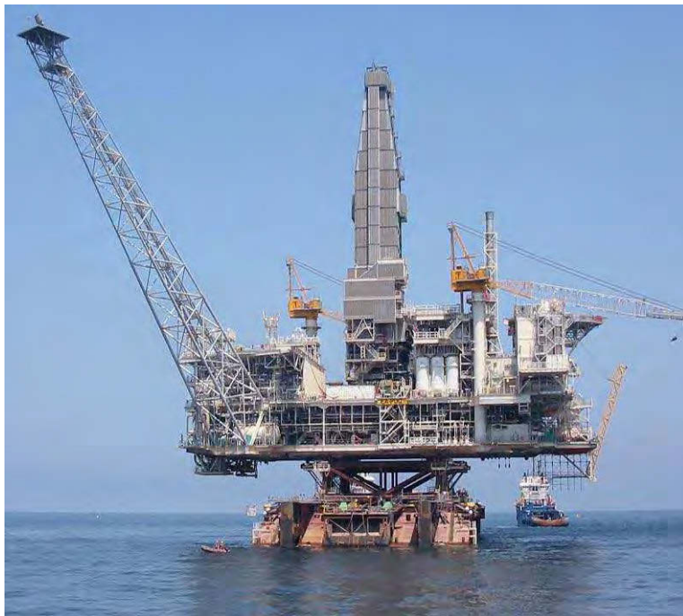
Figure 5.13 EA Platform Topside Onboard STB-01 Barge
