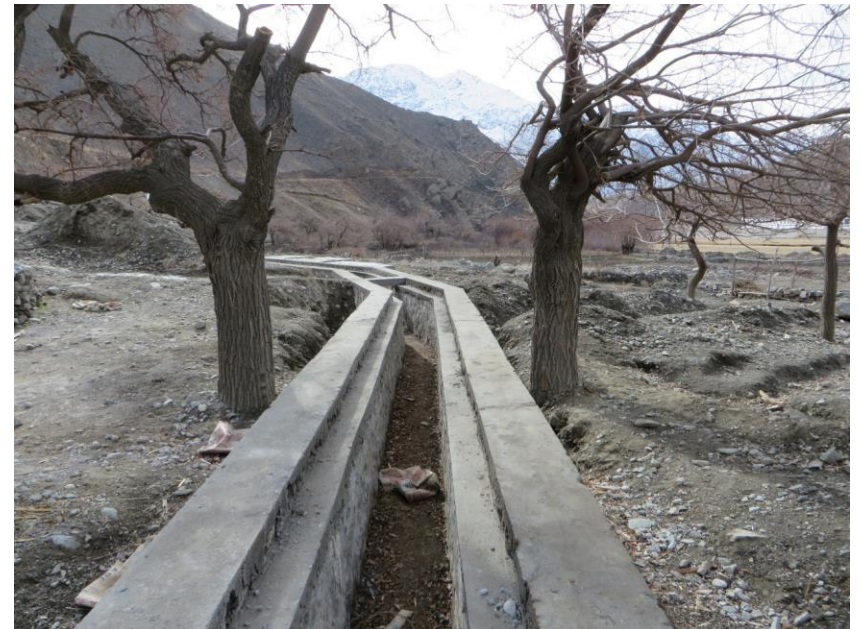
Figure 5 Rehabilitation of Canal- Probil- Panjshir Province
