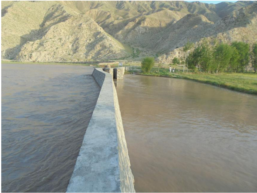
Figure 2 Protection Wall Subproject-Doshi District-Baghlán Province
