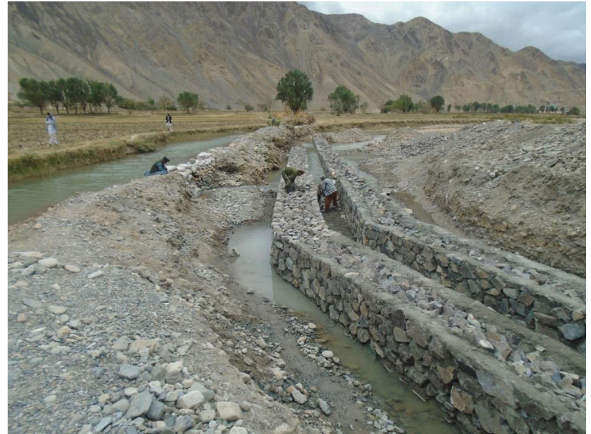
Figure 3 Canal Protection Wall Subproject-Doshi District-Baghlán Province
