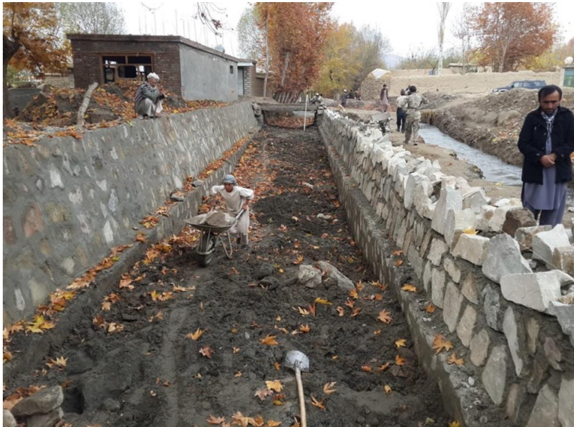
Figure 4 Canal Protection Wall Subproject-Kishm District-Badakhshan Province
