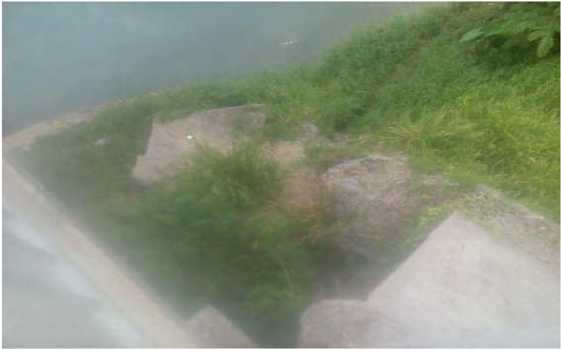
Figure 43. SP12 - Scoured Abutments of Poha High Level Bridge
