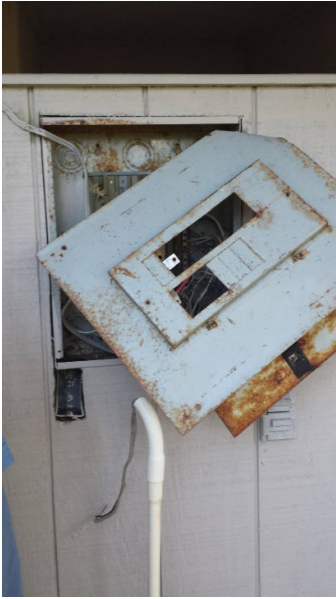
Photo 1: Meter Box blown off from House
