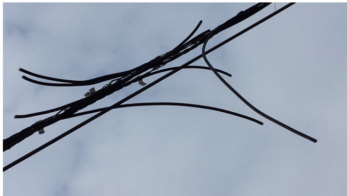
Photo 4: Temporary overhead cable connections installed to restore power, will be easily damaged by high winds.
