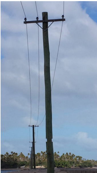
Photo 3: Temporary poles installed to restore power, will not be able to withstand another cyclone.
