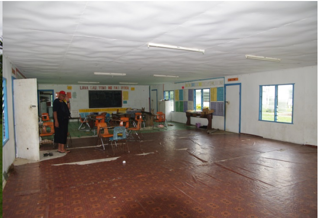
Figure 62 Second Classroom/Hall/Library Building at Mata'aho Government Primary School
