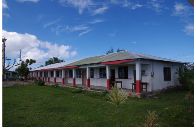
Figure 20 Pangai Government Primary School – Main Classroom Building
