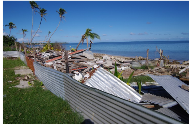
Figure 110 Piled Debris at Tailulu College
