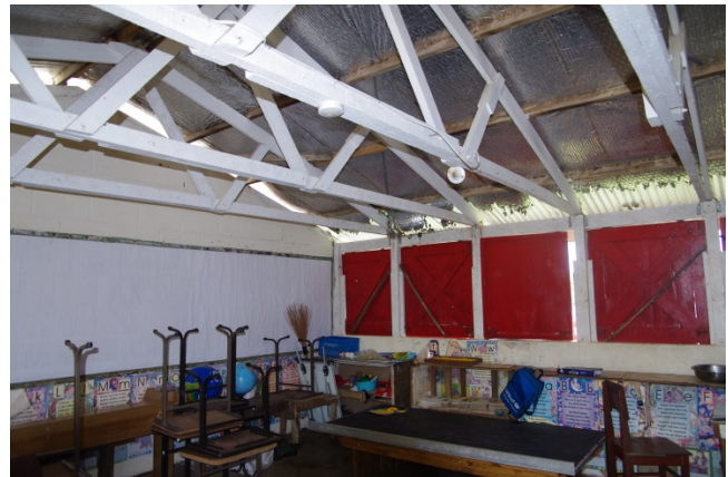
Figure 70 Usable Classroom at Mo'unga'one Government Primary School
