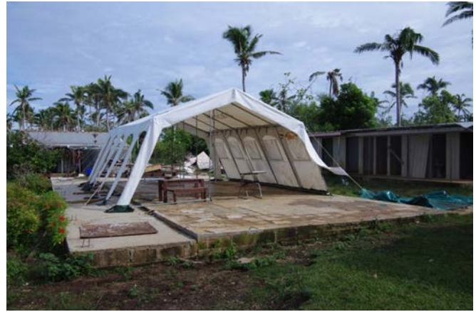
Figure 32 Temporary Teaching Tent at Faleloa Government Primary School
