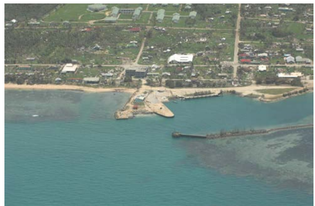
Figure 2 Damage at Pangai Port post Tropical Cyclone Ian (Jan 2014) - Photographs courtesy of the New Zealand Air Force
