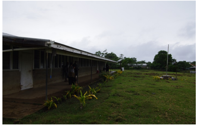
Figure 54 Classroom Building at Lofanga Government Primary School
