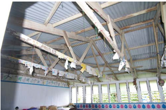
Figure 57 Internal Trusses at Lofanga Government Primary School
