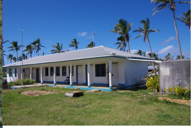
Figure 78 Primary Classroom Block at Ofamo’oni Primary and Secondary School
