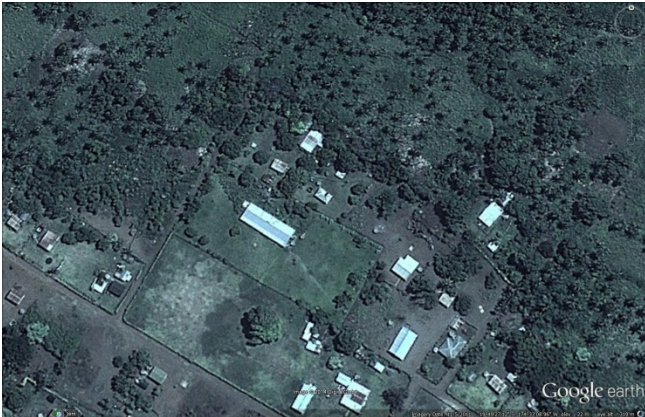
Figure 53 Lofanga Government Primary School - Overview from Google Earth
