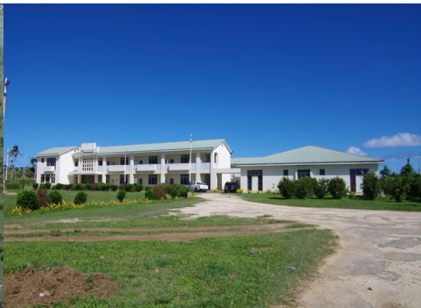
Figure 72 Main Classroom Buildings at Ha'apai High School
