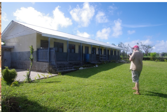
Figure 48 Main Classroom Building Ha'ano Government Primary School
