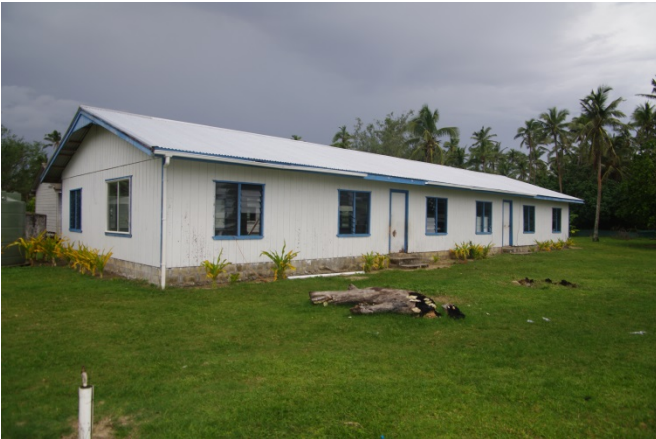
Figure 61 Second Classroom/Hall/Library Building at Mata'aho Government Primary School
