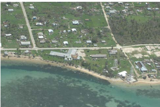
Figure 1 Long Distance shot showing damage at Niu'ui Hospital post Tropical Cyclone Ian (Jan 2014) - Photographs courtesy of the New Zealand Air Force
