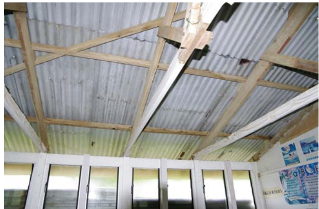
Figure 56 Recycled Roofing Iron with holes at Lofanga Government Primary School
