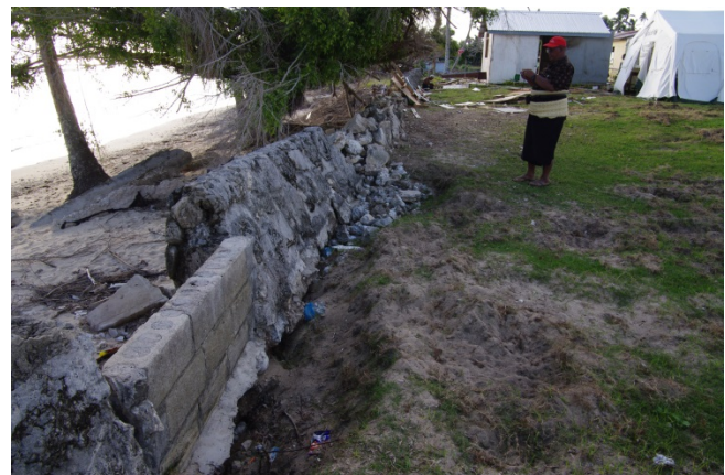
Figure 46 Seawall at Fakakai Government Primary School
