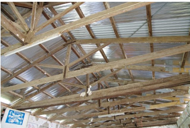
Figure 21 Pangai Government Primary School – Internal Roofing of Main Classroom Building
