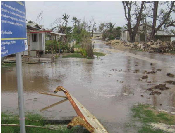
Figure 5 Storm Surge and Sea Flooding associated with Cyclone Kofi
