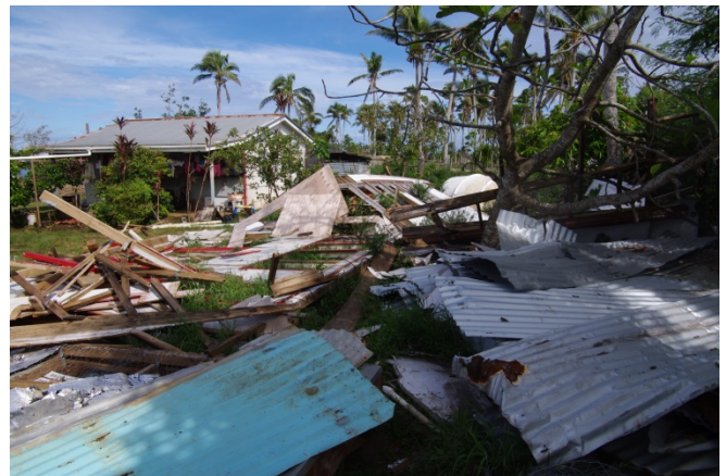
Figure 34 Debris from destroyed building at Faleloa Government Primary School
