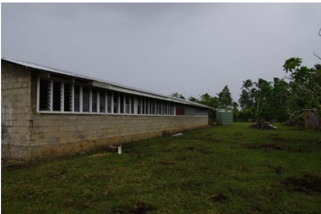
Figure 55 Classroom Building at Lofanga Government Primary School
