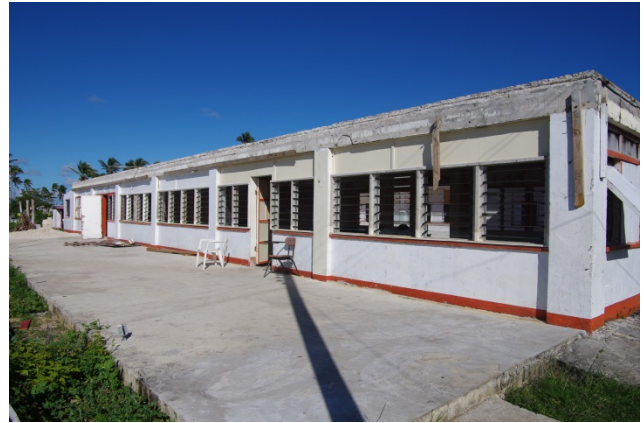
Figure 96 Main Classroom Block at Tailulu College Free Church of Tonga School
