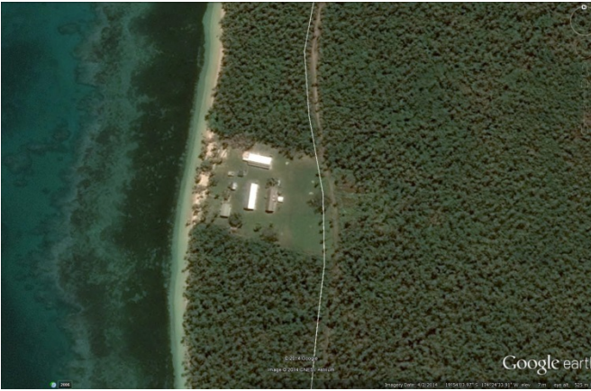
Figure 59 Mata'aho Government Primary School - Overview from Google Earth
