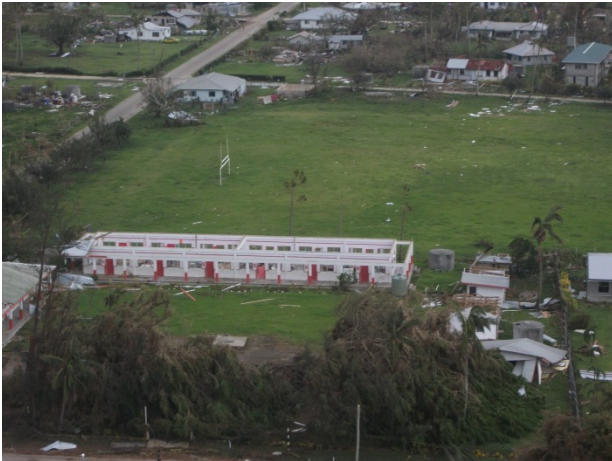
Figure 3 Damage at Pangai Government School post Tropical Cyclone Ian (Jan 2014) - Photographs courtesy of the New Zealand Air Force
