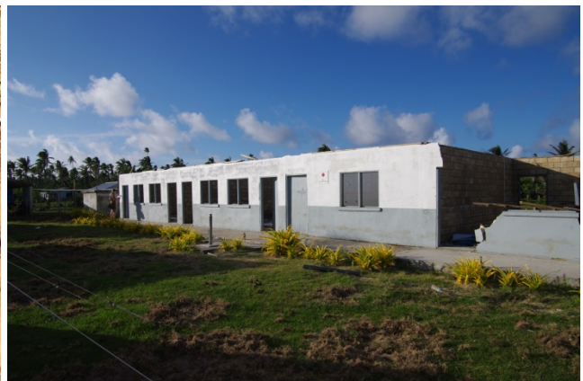
Figure 42 Classroom Block at Fakakai Government Primary School
