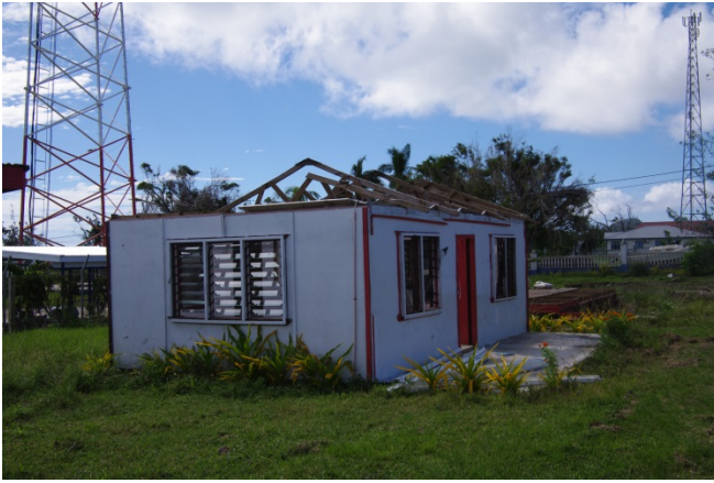
Figure 23 School Office at Pangai Government Primary School
