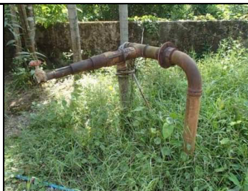
EXISTING TUBE WELL INTAKE
