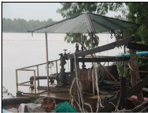
EXISTING RIVER WATER INTAKE FROM THAN LWIN RIVER
