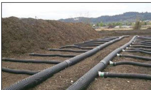
Figure 3-39: Example outdoor composting with aeration pipes system
