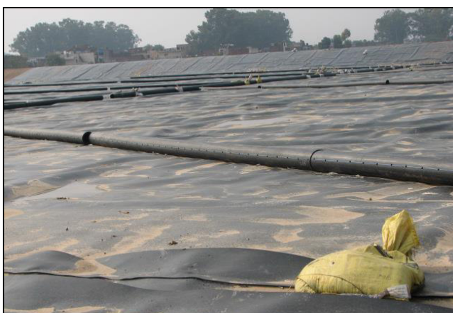
Figure 3-45: Leachate collection system of controlled Landfill
