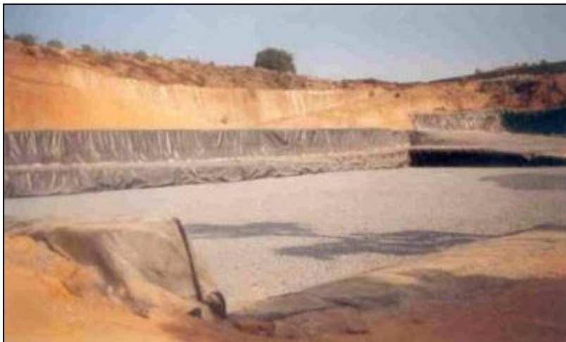
Figure 3-44: Liner system of Controlled Landfill
