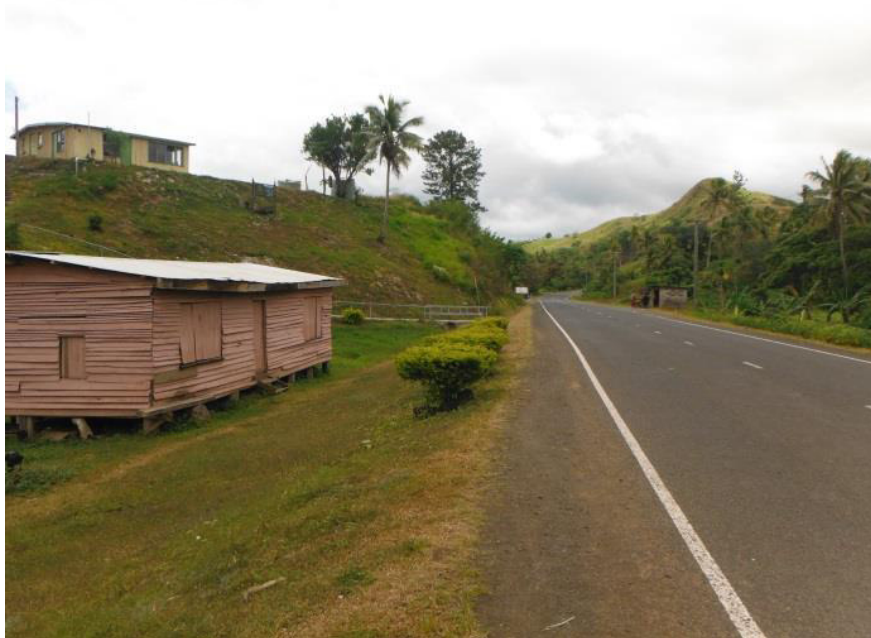
Fig.1 View showing unprotected hazards on outside of curve- site covered under Guardrail Subproject
