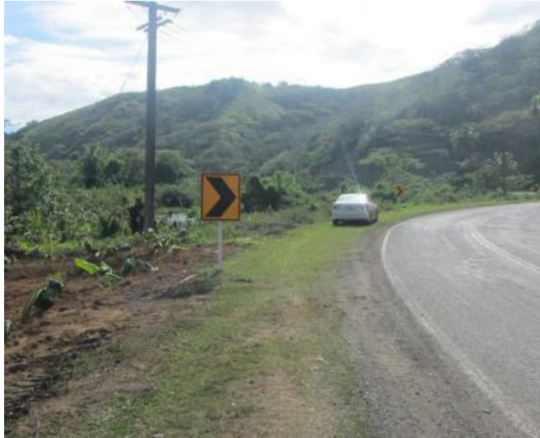
Fig.1 View showing unprotected hazards on outside of curve- site covered under Guardrail Subproject
