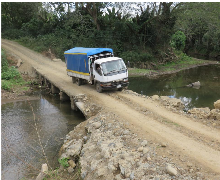
Plate 2: Matewale Crossing. Note the fill in the foreground for temporary repair.
