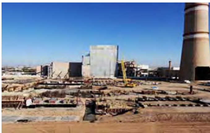
Uzbekistan: Expansion of Talimarjan Power Plant
