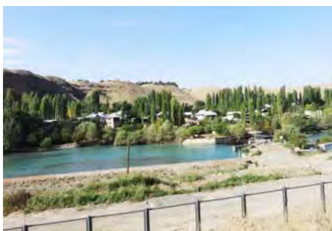
The Kyrgyz Republic: Emergency Assistance for Recovery and Reconstruction project in Osh
