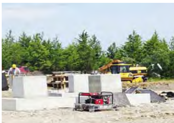
Georgia: Regional Power Transmission Enhancement Project Khorga substation
