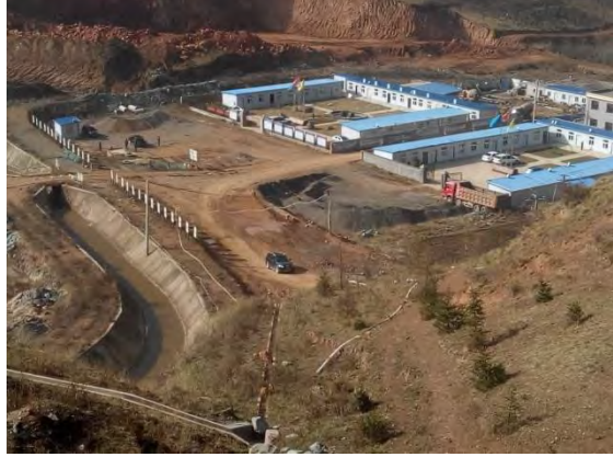
Management station of the Wenzukou Reservoir
