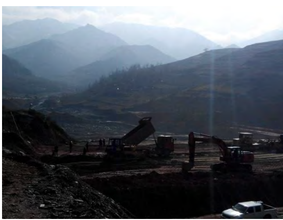
Construction site of Wenzukou Reservoir
