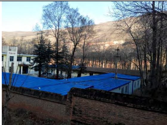
Management station of the Fatai Reservoir
