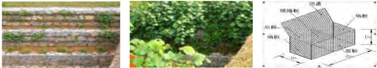
Figure VI.1: Metal gabion retaining wall
