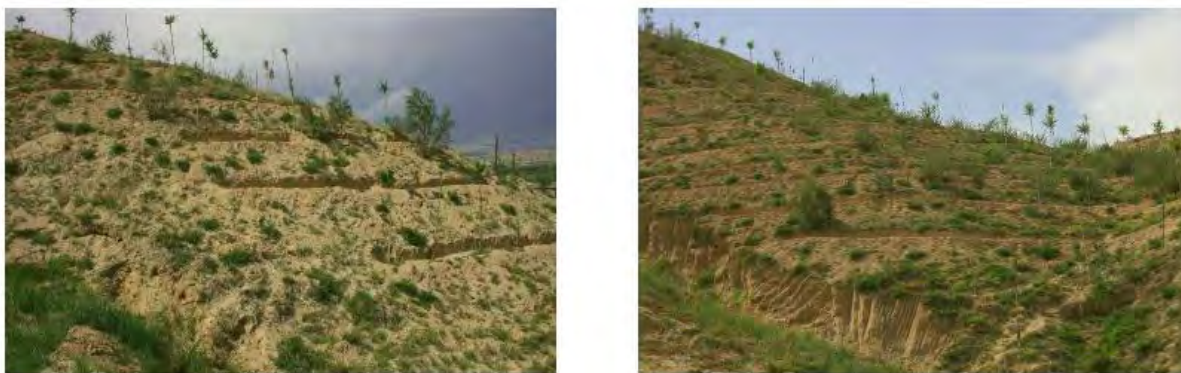
Figure V.2: Slope stabilization in compliance with Soil and Water Conservation Law (2010)
