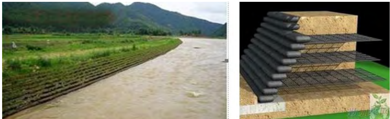
Figure VI.2: Green Dam eco-bags retaining wall
