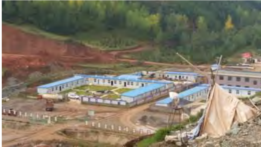
Figure V.3: Site of Wenzukou WTP
