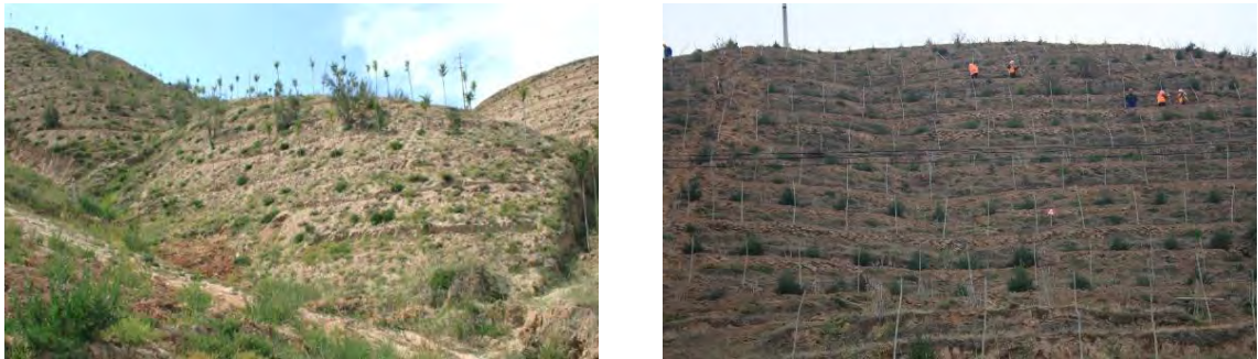
Figure IV.23: Existing Mountain Edge Stabilization and Revegetation
