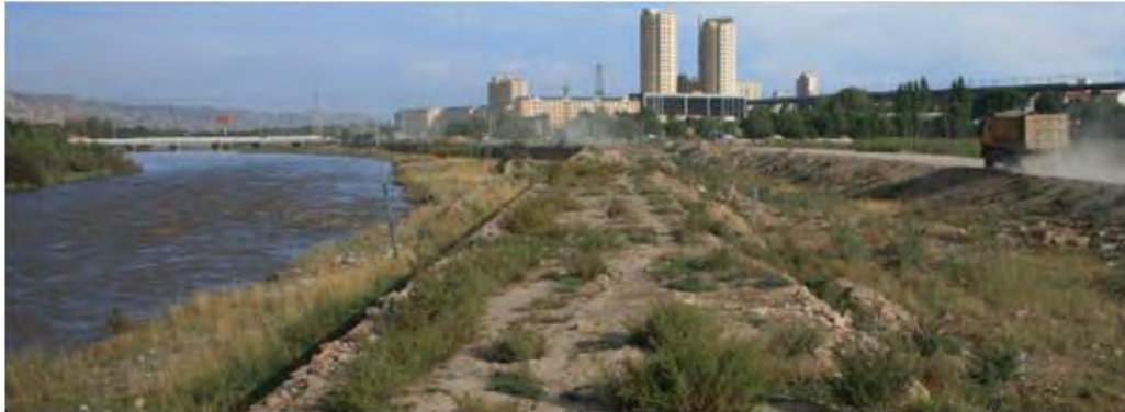
Figure IV.15: Right Bank near Haidong showing some riparian vegetation below the flood embankment and the area between the top of the wall and the adjacent road covered in weeds.
