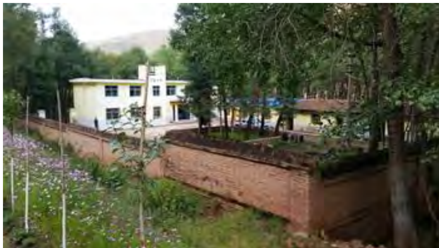
Figure V.4: Site of Fatai WTP
