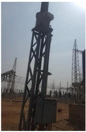
220 kv CVT to be replaced
