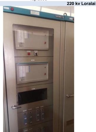
Existing Fault Recorder report out of order to be replaced
