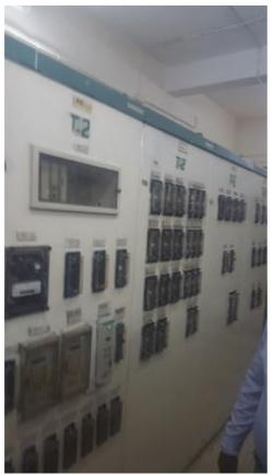
Existing Over Voltage Relay to be replaced
