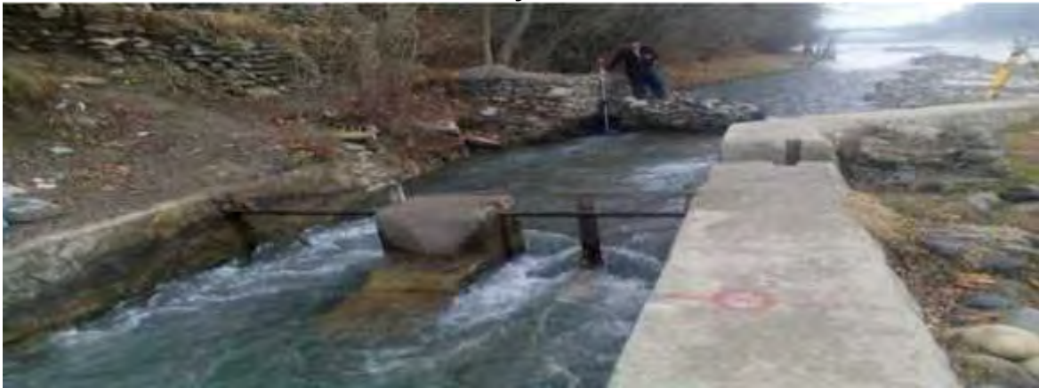
Photo: RSP Seyaab, Headwork
