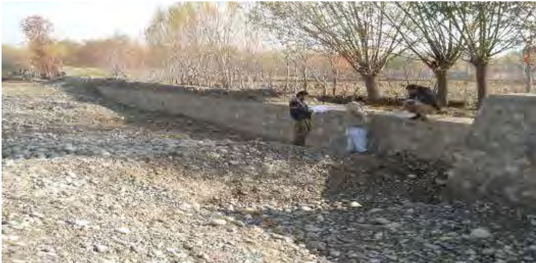
Photo: RSP Sharawan, Bank Protection Near Headwork
