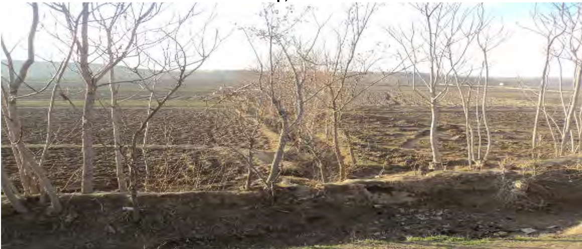
Photo: RSP Laqi, Nematullah Canal
