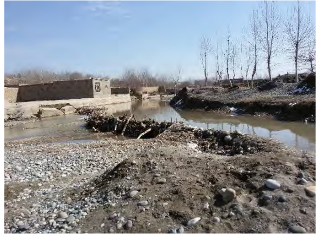
2. Offtake and weir Baghak
