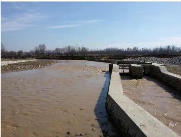
3. Rehabilitation of existing offtake Konchi
