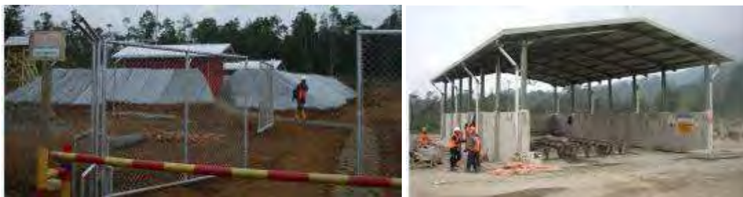
Figure 2.4: Construction base camp and Temporary Drilling Cutting Storage
