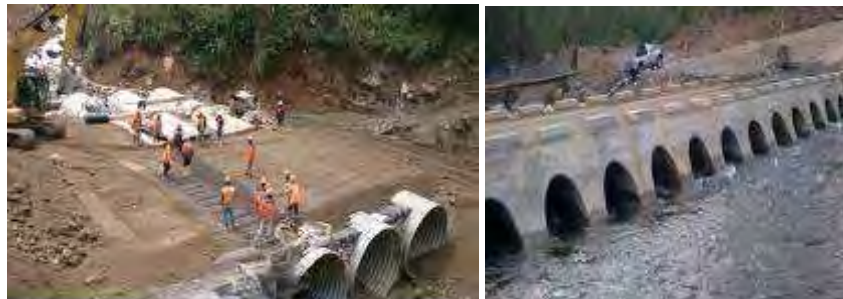
Figure 2.5: Construction of Bridge at Endikat River
