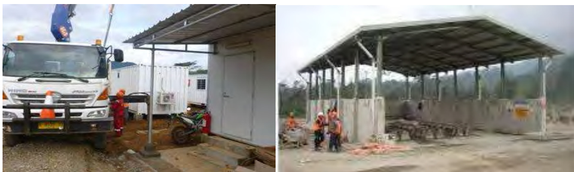
Figure 2.4: Construction of Base Camp and Temporary Drilling Cutting Storage
