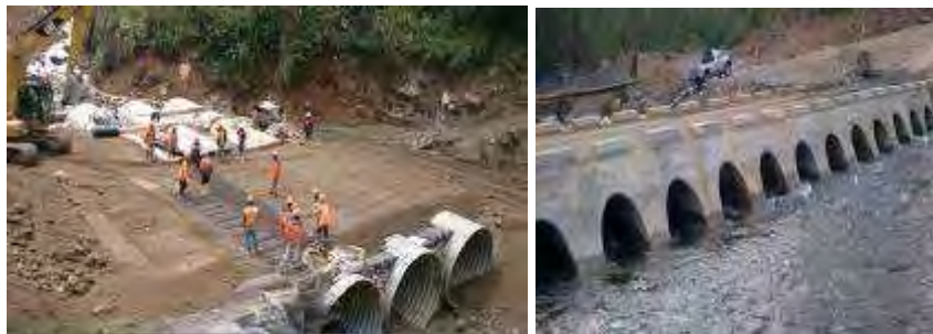
Figure 2.5: Construction of Bridge at Cawang Tengah River and Endikat River
