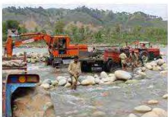
Extraction of Gravel and Sand from River Bed
