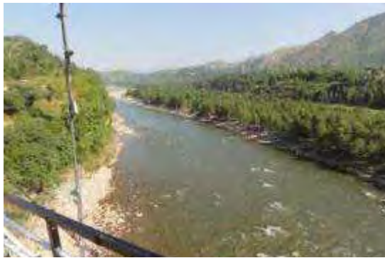
a. Upstream of Kallar Bridge
