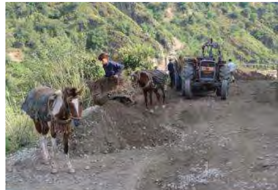
Sand Dumping on Road Side near confluence of Poonch River and Ban Nullah
