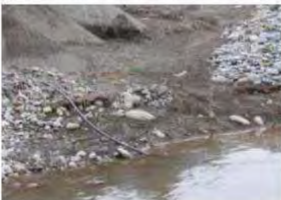
Water Pumping from River
