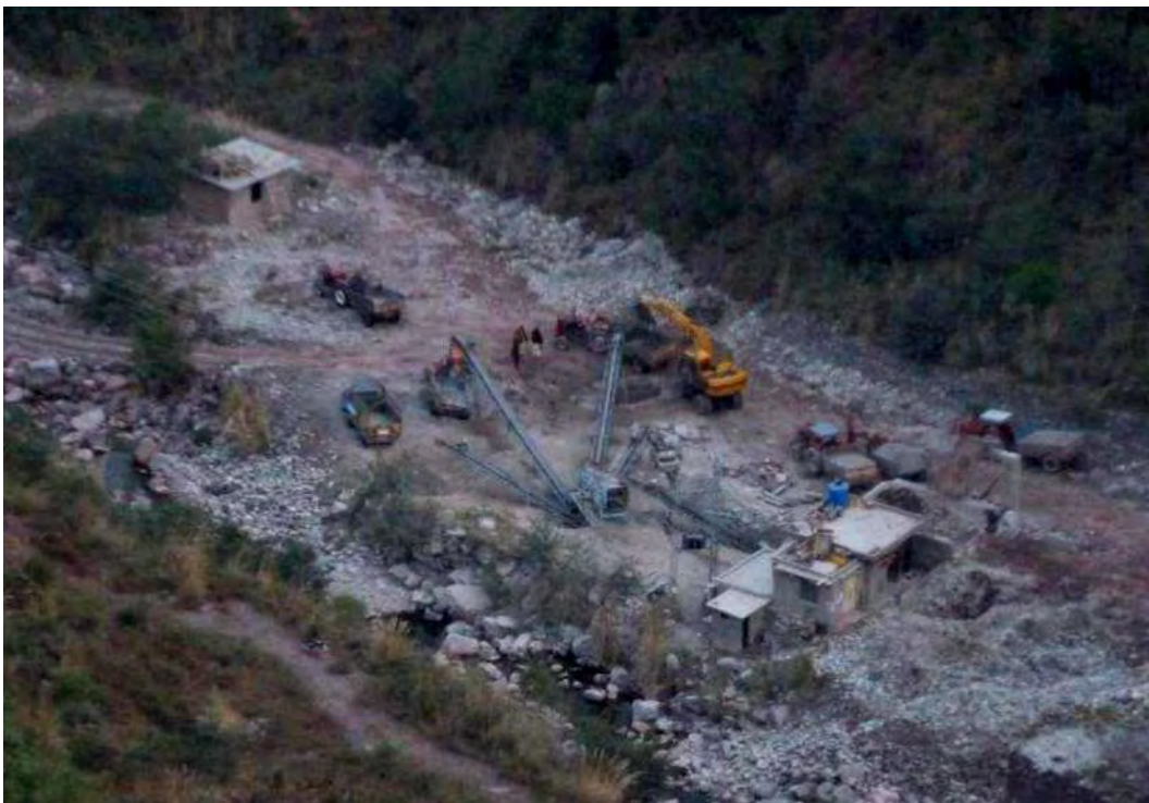
Figure 5-30: Mining Operation in the Bed of a Tributary where Extraction of River Sediment for Construction and Road Building is Degrading the Instream and Riparian Habitat of these Reaches
