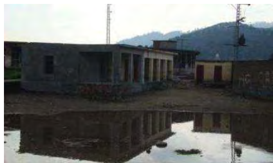
Lack of proper drainage infrastructure in Kotli
