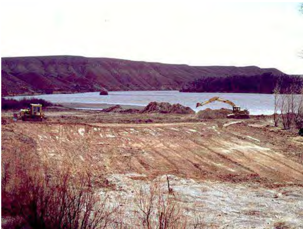
Figure 3-4 Restoration of floodplain connectivity on the Green River, Utah. Levee breaches were done by excavating a “notch” in the levee or by lowering the existing levee height. Some breaches were narrow channels which backfill slowly, while others had large portions of the levee removed to allow the river current to push water into the site. http://wildfish.montana.edu/Cases . Accessed 27.03.2104
