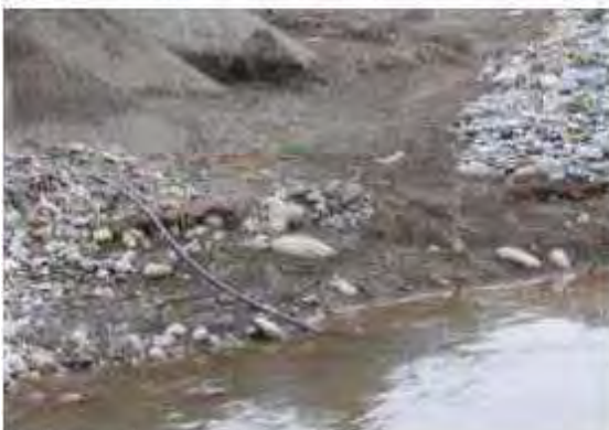
Water Pumping from River
