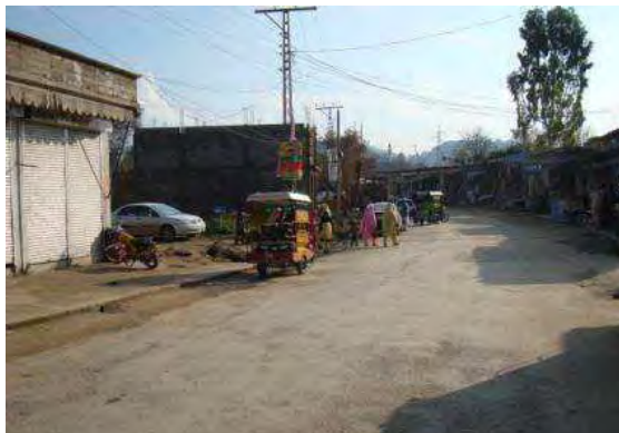
View of blacktop road in Rajdhani
