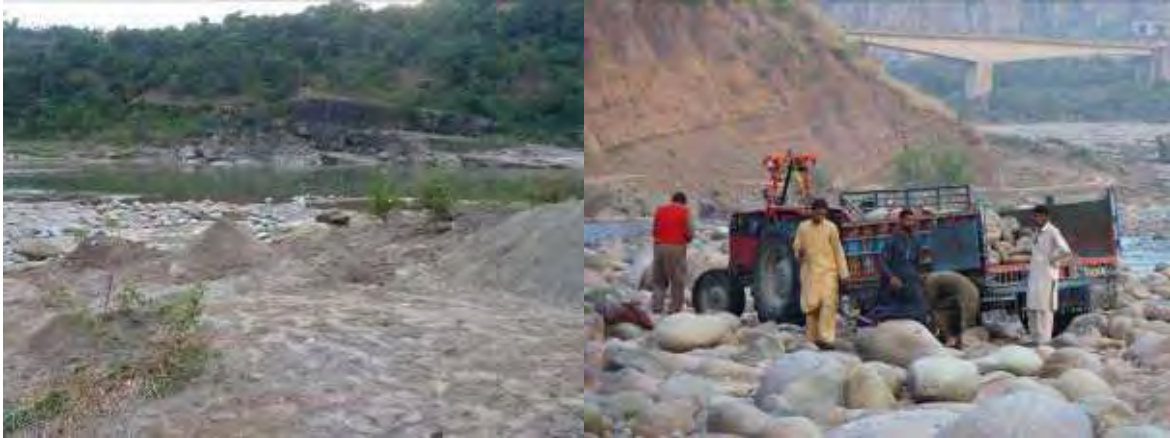
Figure 1-1 Extraction of fine sands (left) and cobbles (right) on the Poonch River near EF Site 2
