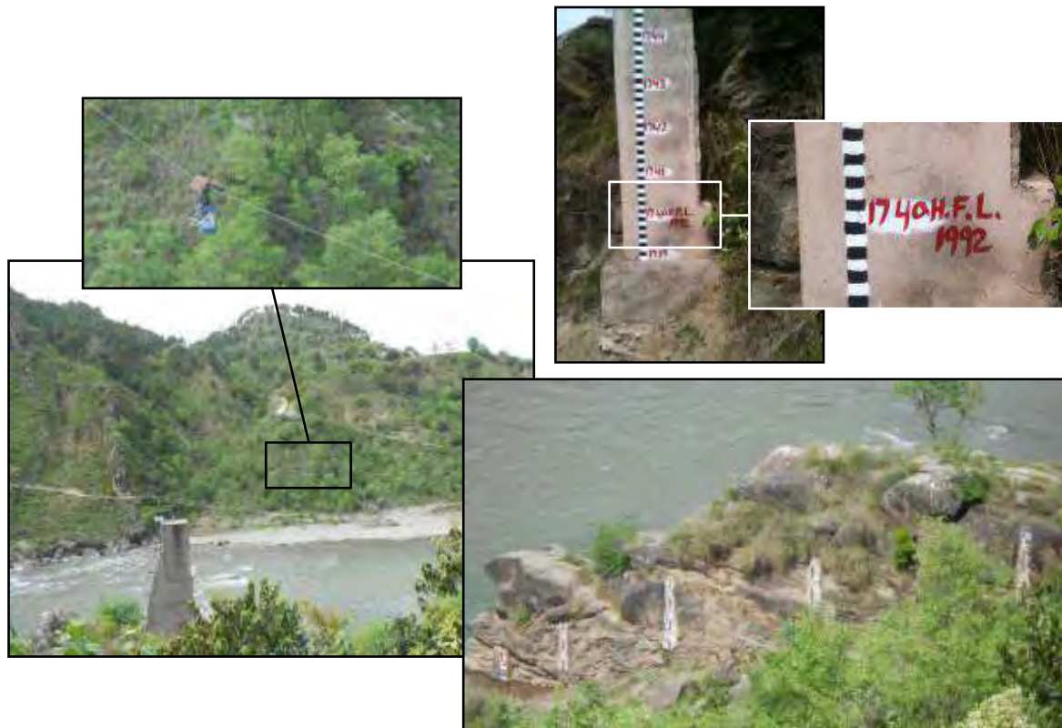
Figure 2.11 Photographs of the Rehman Bridge Gauging Station, located c. 130 m below the confluence of the Poonch River and Ban Nullah. Note the 1992 High Flood Level (HFL) of 1740 ft amsl (source: Mr Yasir Abbas, NESPAK)
