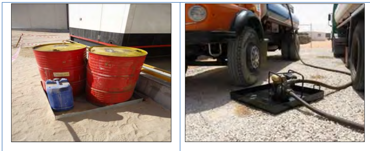
Figure 11.4: Drip Trays under Fuel Hoses and Drums Stored Temporarily
