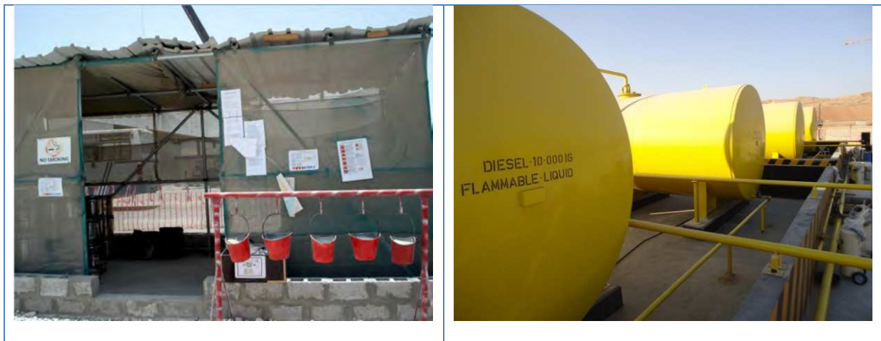
Figure 11.2: Hazardous Storage Area and Diesel Tanks Containment Basin
