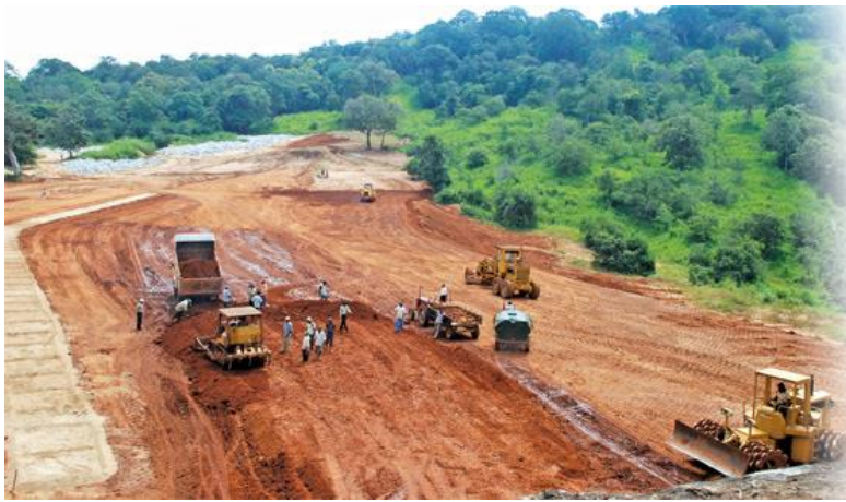
Final phase of Mahaweli Development Scheme underway
