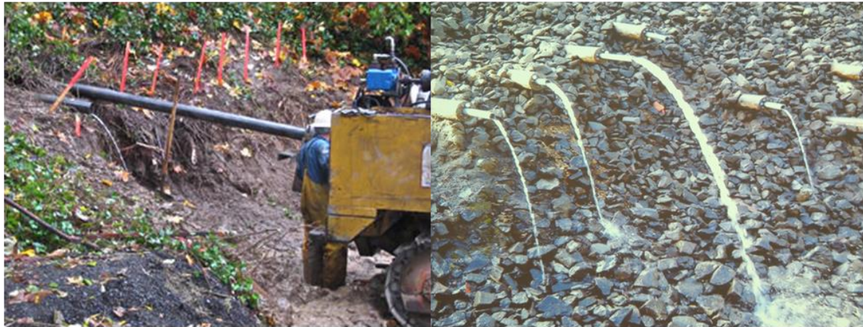
Left: Installing Horizontal drains on slopes and right: horizontal drains in operation
