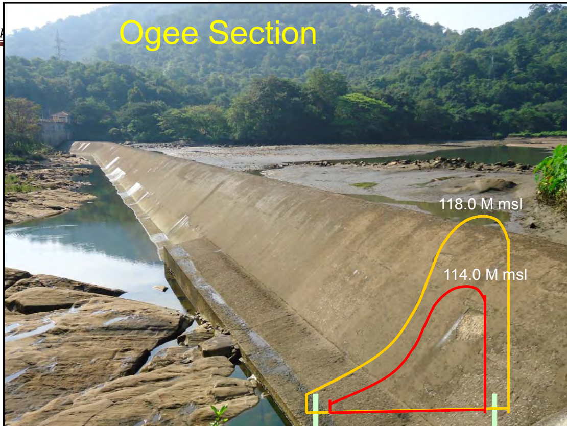
Figure 6 Existing Anicut Indicating the proposed Changes
