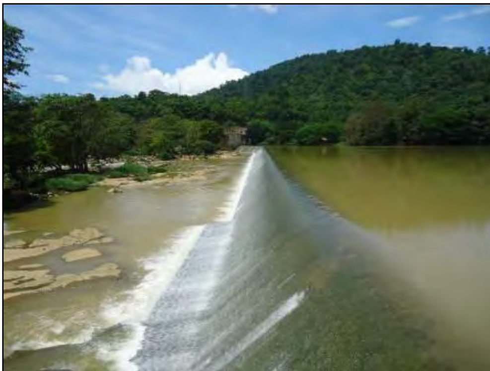
Figure 13. Spillage of water over the Minipe Anicut during the peak power generation period of the day at Rantambe power house.
