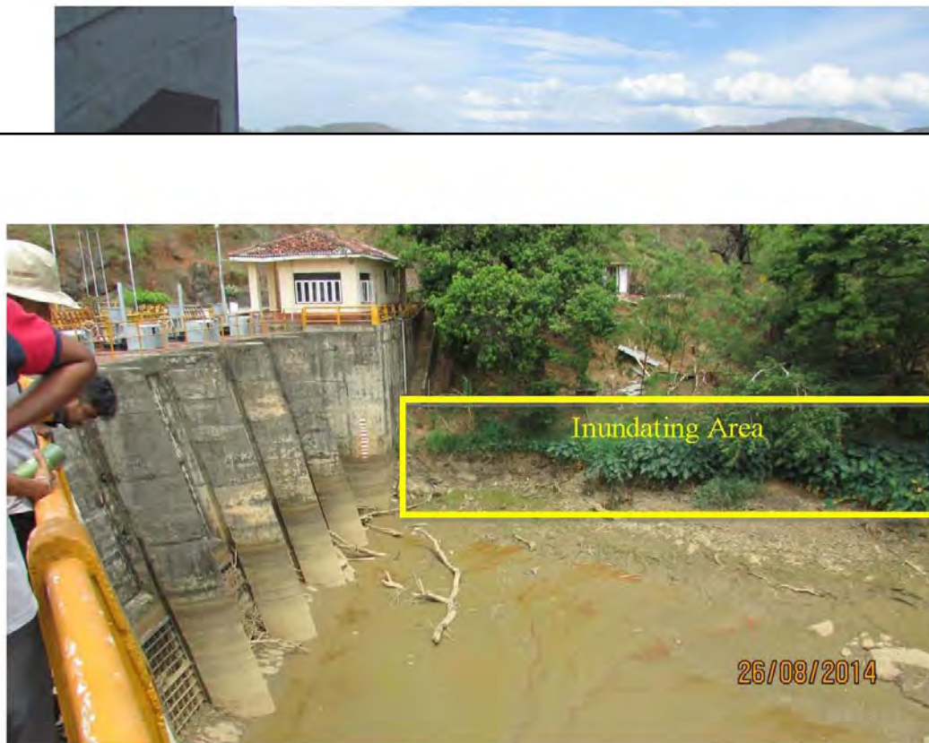
Figure 08. Right Bank and Gate of the RB Canal with Road embankment which should be protected
