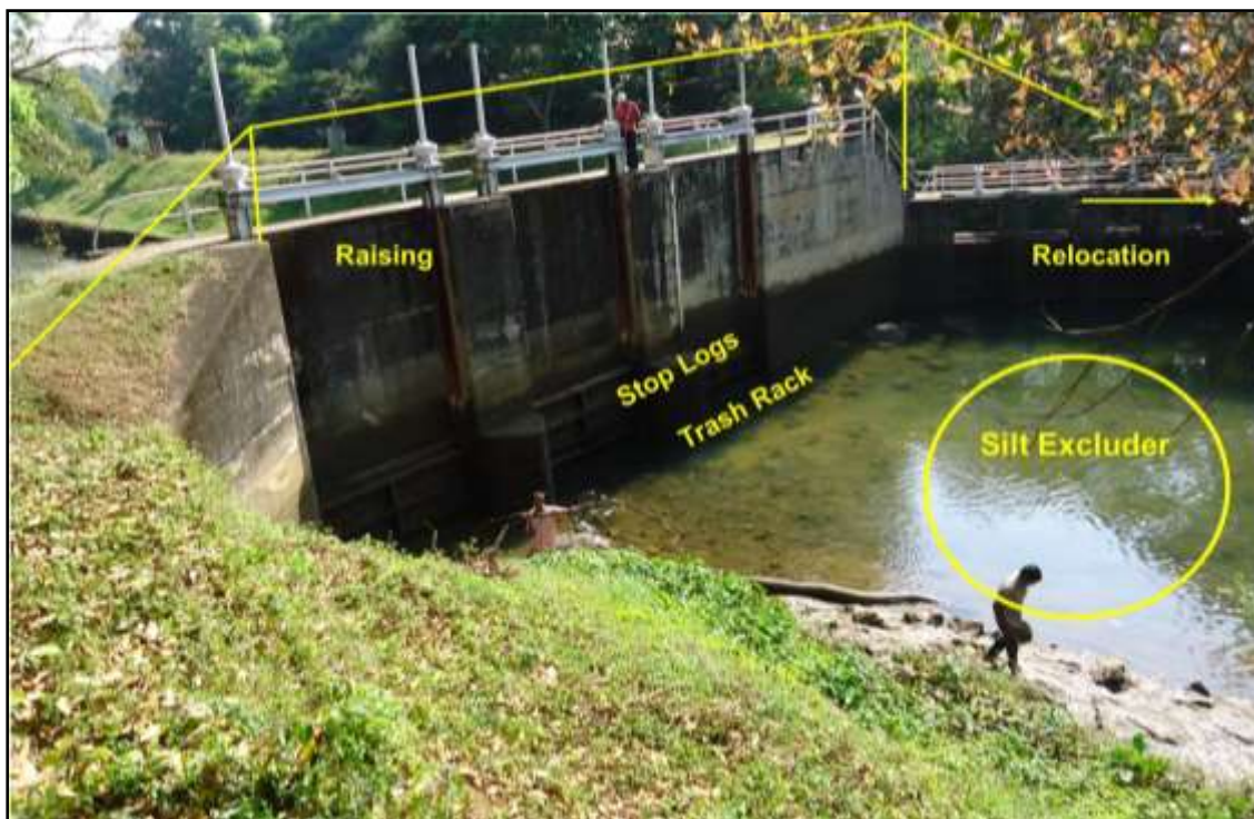
Figure 7 Proposed changes to the LB Sluice and Silt Excluder
