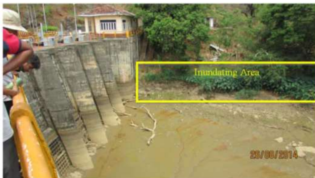
Figure 08. Right Bank and Gate of the RB Canal with Road embankment which should be protected
