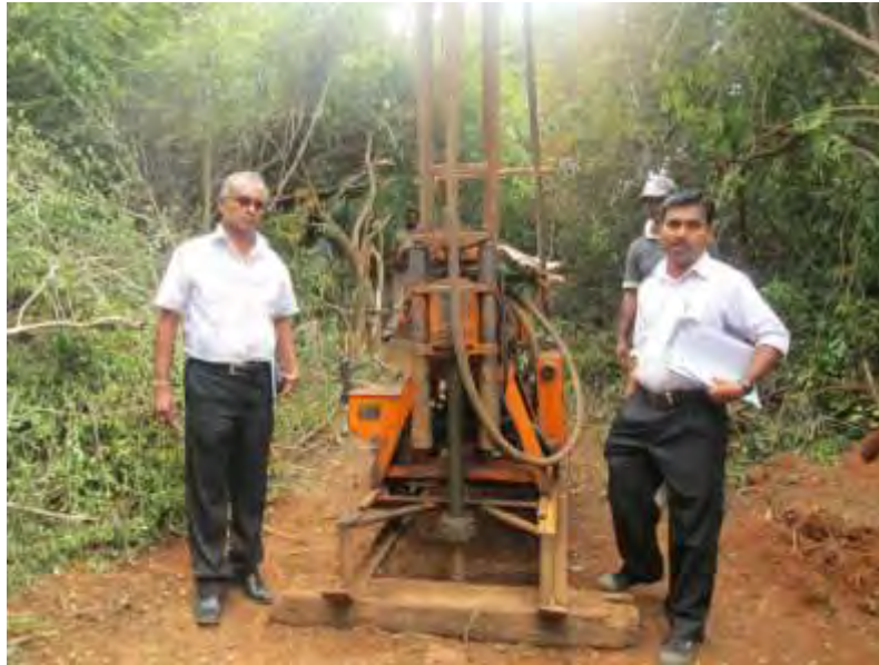
Plate 3.2 Drill hole location at 17+770km - above Madatta wewa
