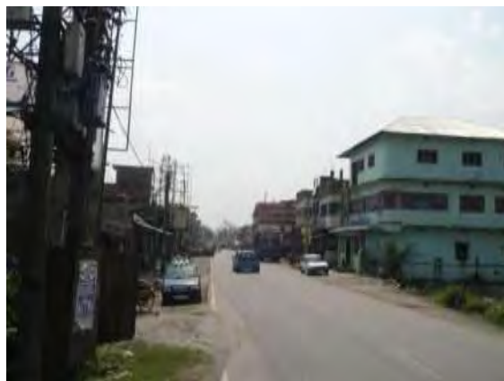
New Hasimara - Built up section
