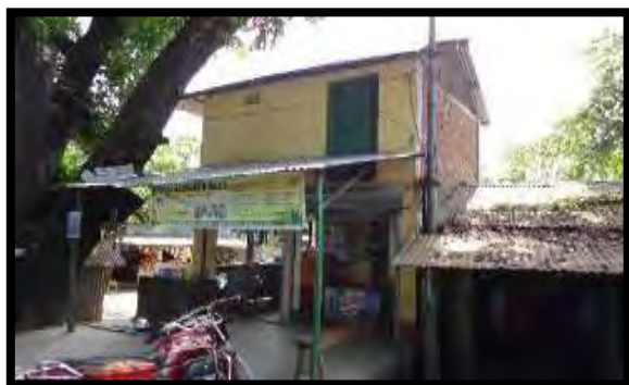
Commercial DP-Asset No.542 in Uttardanga para Km 49.587 - Offset 9.8m - RHS
