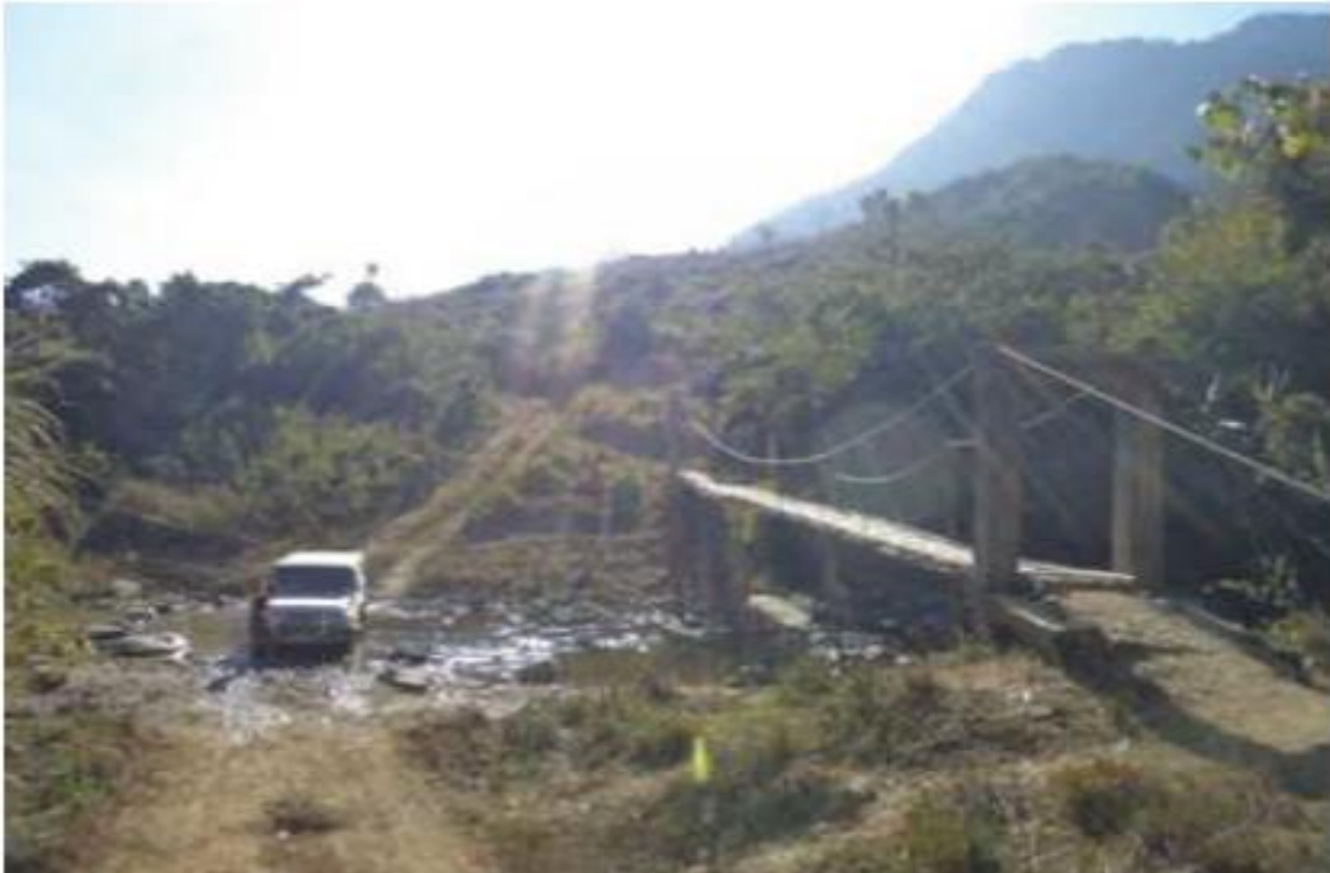
Iring River at km 61+058
