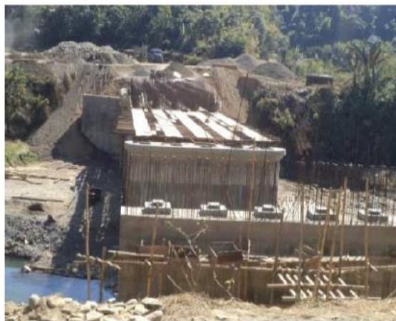
Under construction Bridge at Km 81+075 over Irang River
