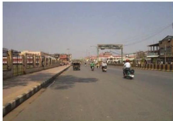
Existing Fly Over approach at Km 0+500
