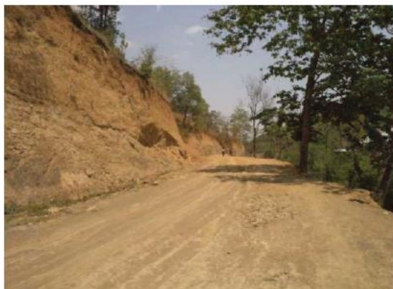
Existing track near Kangchup Village at Km 16
