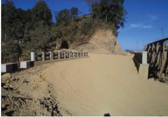
Bridge at Km 108+680 near Tamenglong
