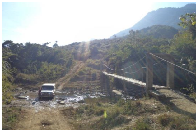
Image 3: Iring River at km 51+900 on Project Riad in hill section
