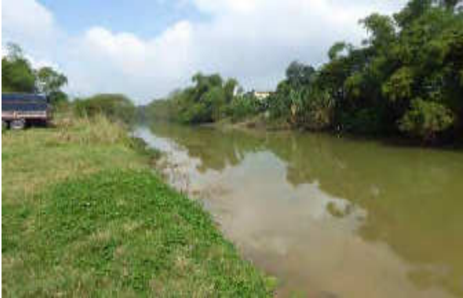
Figure 6. Section of Ke Van river to be dredged & embankment (left) stabilization.
