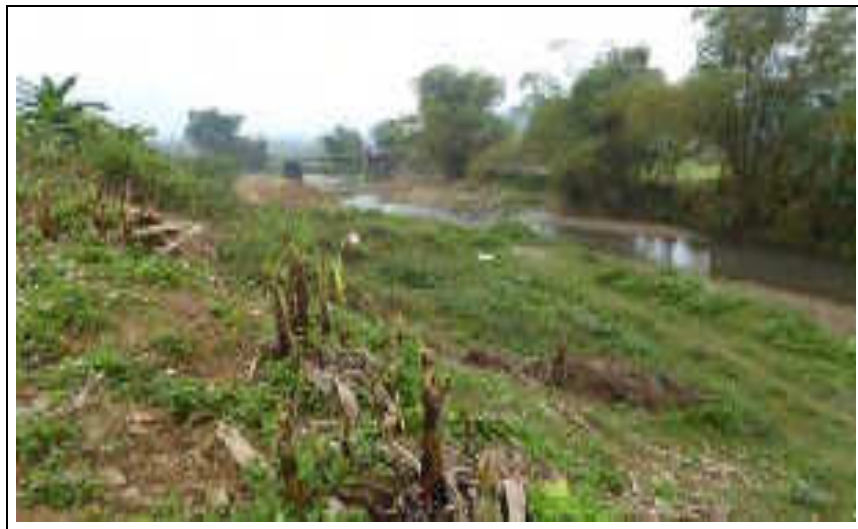
Figure 38. Embankments of Me stream to be rehabilitated
