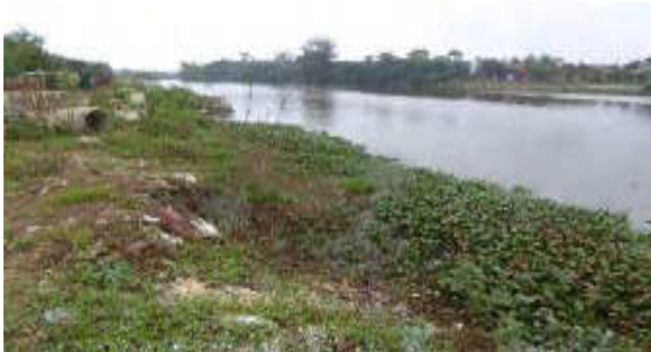
Figure 14. Embankment of Nhu Y river to be rehabilitated.
