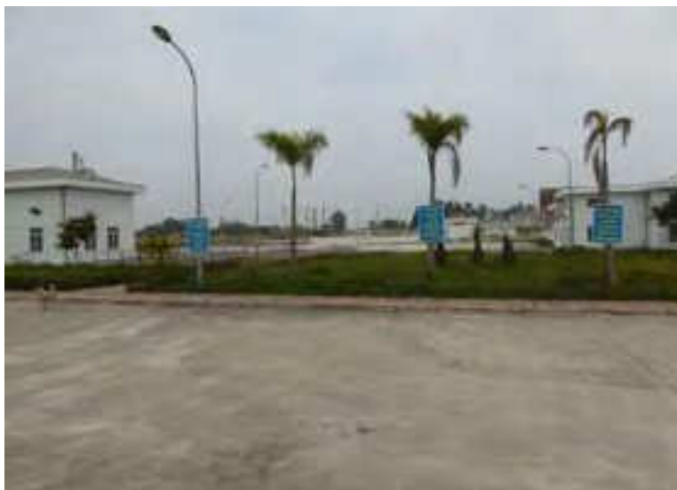
Figure 54. Existing JICA WWTP
