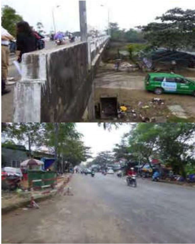
Figure 25. Vy Da bridge an Pham Van Dong approach road
