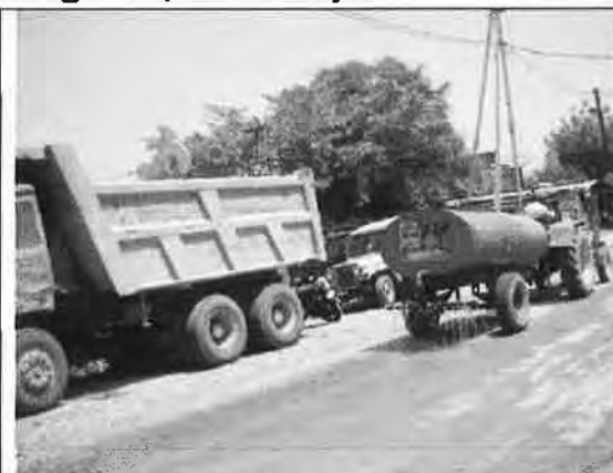
View of water sprinkling at construction site at km4.400.
