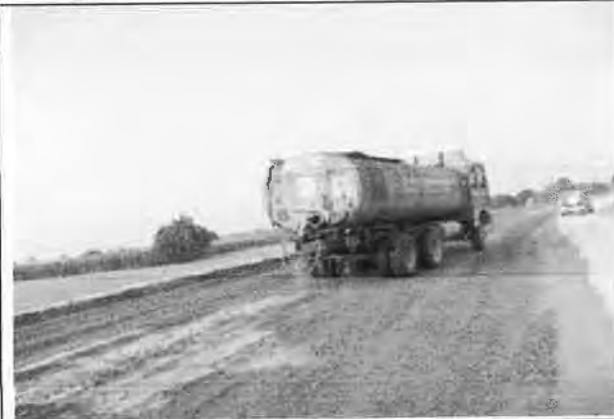
A view of water sprinkling at site for mitigation of dust pollution
