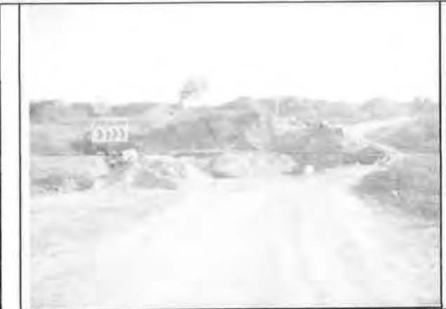
View of safety measures at cross drainage structure construction site (Diversion board and safety tapes)
